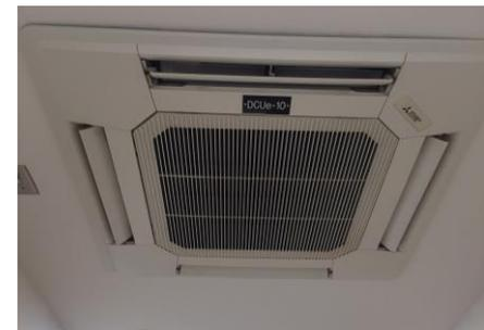
ASHPs use a refrigerant loop to extract and move heat between spaces. Systems can provide both heating AND cooling.
