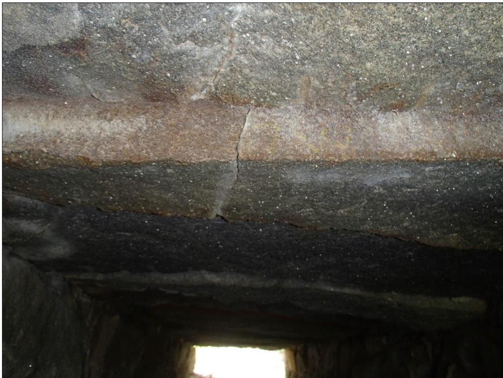
Photo 12 Looking North: Crack in Roof on South Side of West Span
