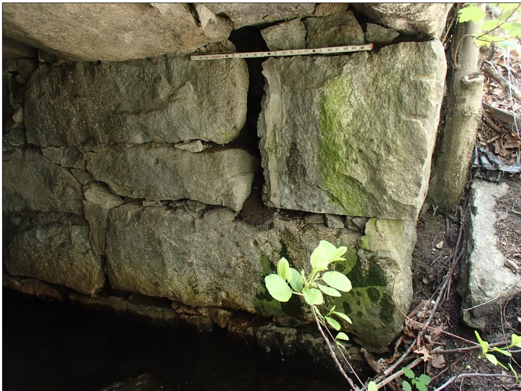
Photo 10 Looking West: Northwest Corner Voids
