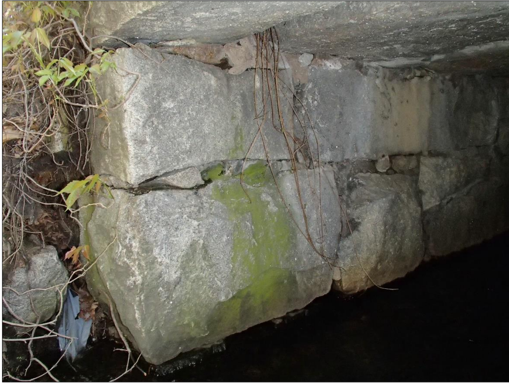
Photo 11 Looking East: Northeast Corner Voids
