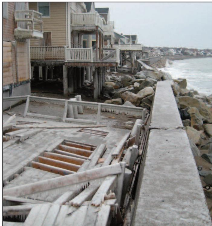
***Decks, stairs, siding, and other parts of these buildings were damaged by waves and flooding in a nor'easter. Repairs to these houses will require permits under the State Building Code and Wetlands Protection Act regulations, and possibly the local wetlands bylaw.***
