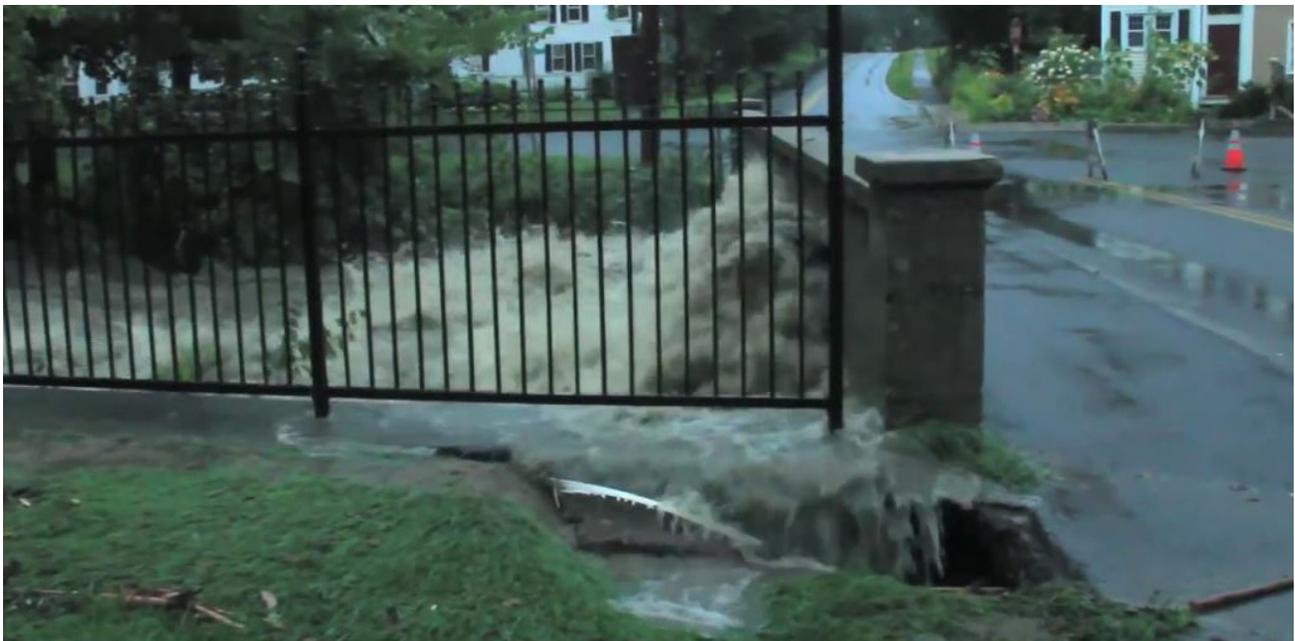
*Above: The North St. bridge during Hurricane Irene in 2011. The river's water level reached a record-breaking 16.42' during that storm, and its velocity was recorded at over 7,000 cubic feet per second. A new stone cap on the wall at Meekins Library likely prevented the river from damaging the street, unlike in 1936 when the river spilled its banks and destroyed the street. (Source: Folktography by Tom)*
