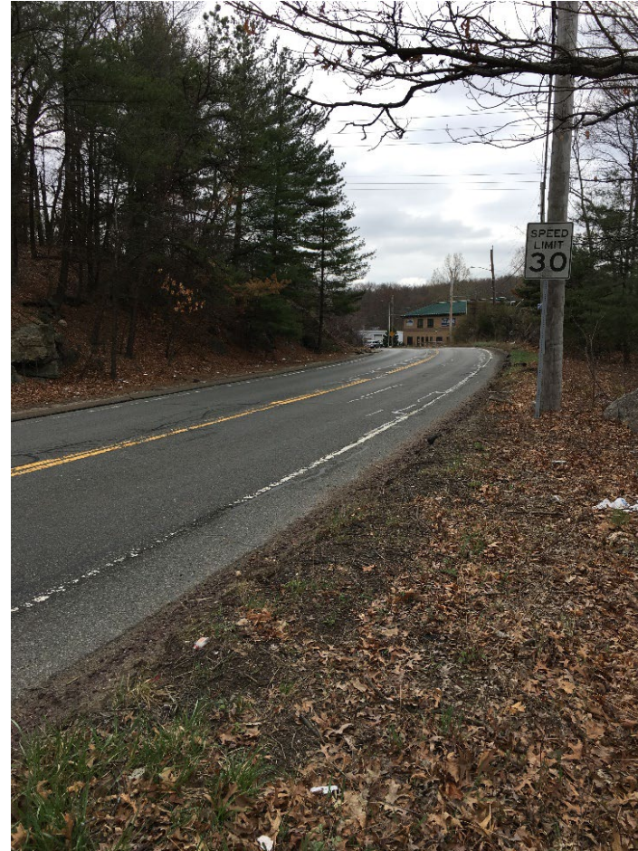
Narrow shoulder, lack of sidewalks, and limited sight distance
