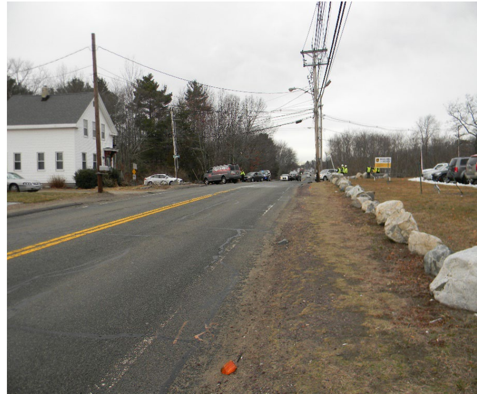
Narrow shoulder, deficient pedestrian accommodations, high crash rate, and sharp crest curve limits sight distance
