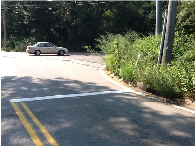
Figure 1 – Hazard Vegetation at intersection of Concord Street and Woburn Street Hazard vegetation obstructs site distance at critical intersections.
