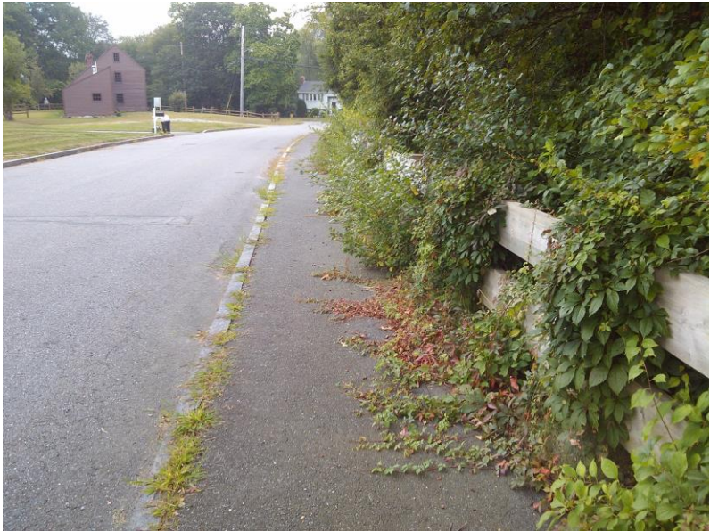
Figure 3 – Nuisance and Invasive Vegetation on Marion Street Nuisance vegetation creates a public safety hazard to workers and pedestrians.
