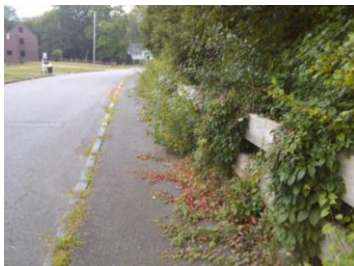
Marion Street – (Prior to implementing VMP)
