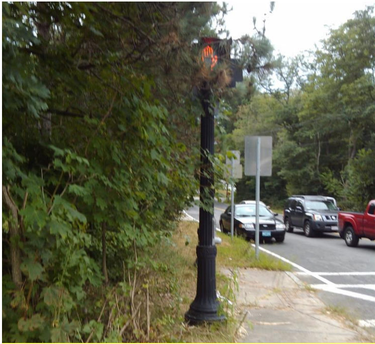
Figure 4 –Hazard Vegetation blocking a traffic signal at Woburn Street and Salem Street Hazard vegetation obstructs critical utilities.
