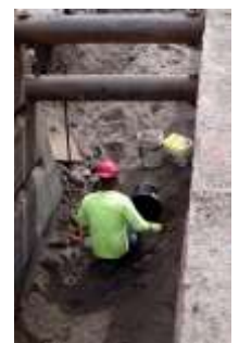
Installation of a new water main on Winthrop Shore Drive
