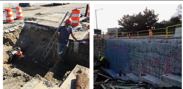
Left: Installation of a new water main Right: Seawall repairs in Highlands area
