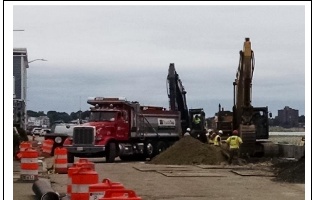
Excavation for new storm drainage system in Winthrop Shore Drive. 7/14/17
