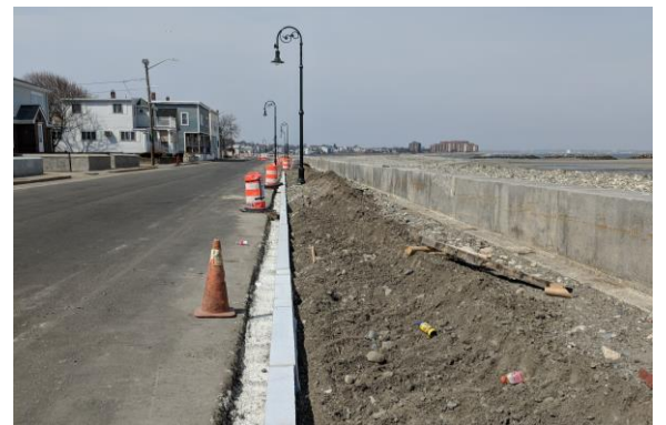
Curb installation north of Beacon Circle.
