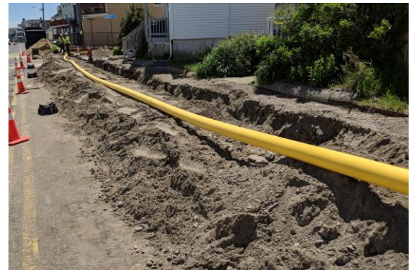
New gas pipe near Locust Street.
