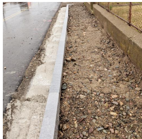
New granite curb has been installed and the gravel base is ready for the new concrete sidewalk to be poured.
