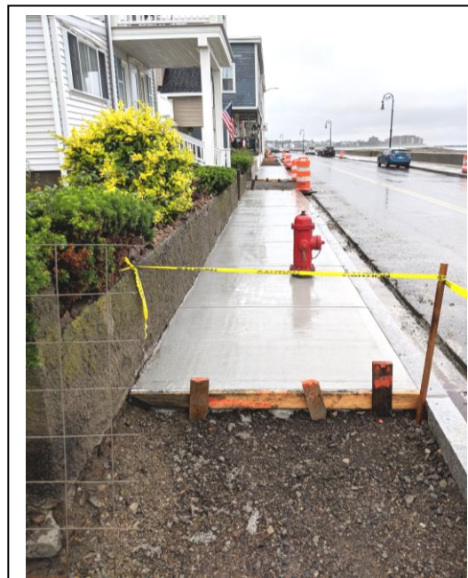
New concrete sidewalks are poured in alternating sections.
