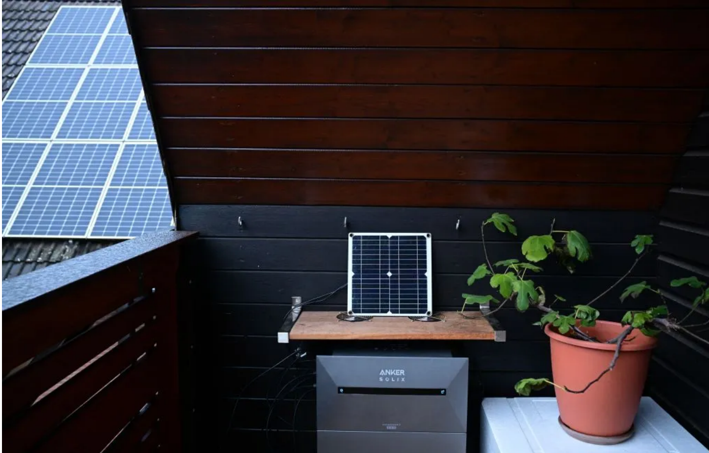
Balcony solar systems feature one or two small photovoltaic panels and a microinverter and generate enough power to charge a laptop or power a small fridge. PHOTOGRAPH: TOBIAS SCHWARZ/GETTY IMAGES
