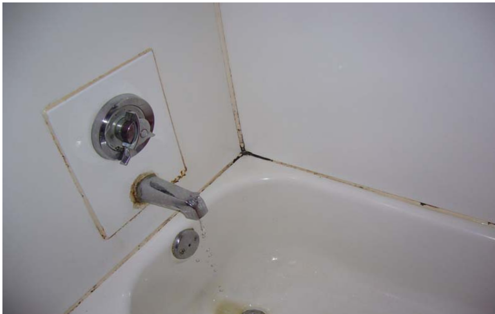
200-1 Development, 83 Creston Avenue - Mold and Mildew in Bathroom
