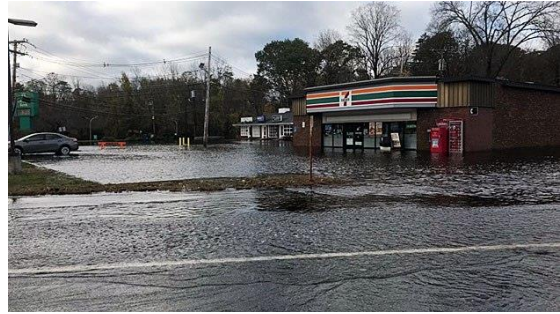
Figure 2. Flooding at Four Corners Source: CBS Boston, 2017
