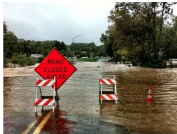
Figure 6. Woburn exit off Route 128 closed. Source: Patch, 2016
