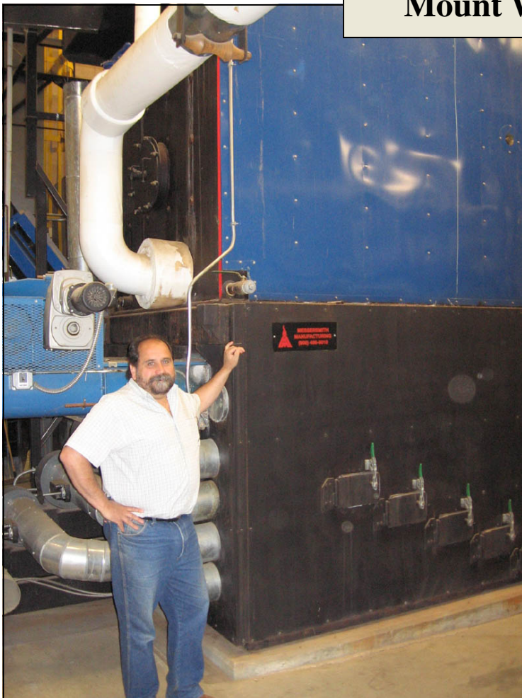
Rob Rizzo, Director of Renewable Energy Studies at Mount Wachusett Community College stands next to the 8 MMBTU wood fired boiler that replaced an expensive electric heating and cooling system.
