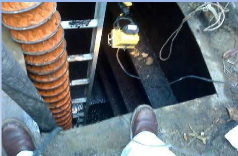
Ventilation hoses provide air and exhaust toxic vapors during permit required confined space entry. A guardrail would also be necessary to protect workers from potential falls.
