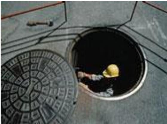
Many workplaces contain areas that are considered "confined spaces" because while they are not necessarily designed for people, they are large enough for workers to enter and perform certain jobs. A confined space also has limited or restricted means for entry or exit and is not designed for continuous occupancy. Confined spaces include, but are not limited to, tanks, vessels, silos, storage bins, hoppers, vaults, pits, manholes, tunnels, equipment housings, ductwork, pipelines, etc.
