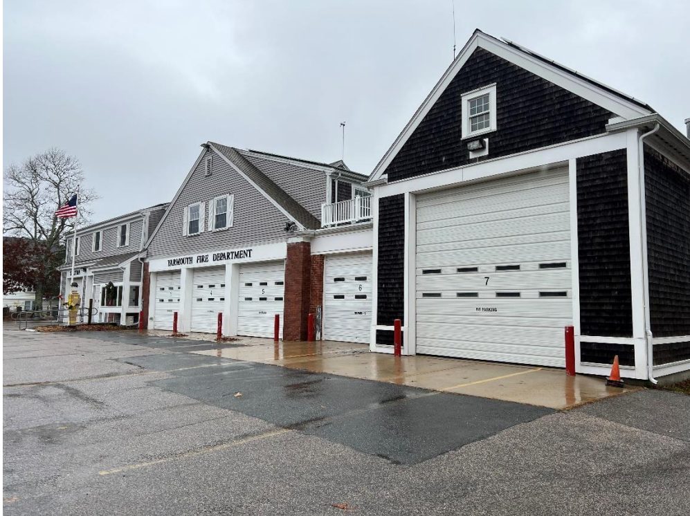
Old Main Fire Station
