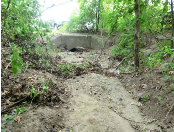
Existing culvert, 90%-filled with sediment.
