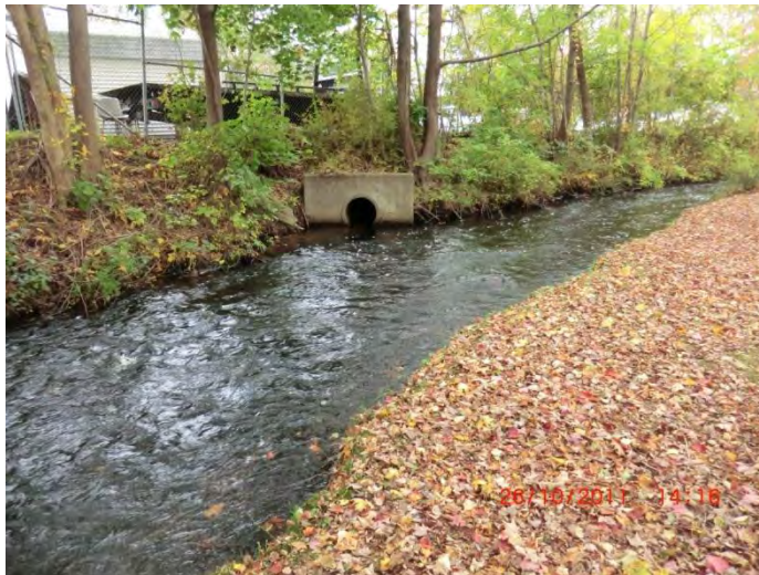
Storm water outfall to Rumford River below Fulton Pond.
