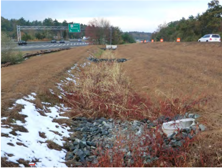
Ex-BMP-2. Dry Water Quality Swale.
