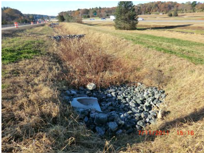
Ex-BMP-1. Dry Water Quality Swale.
