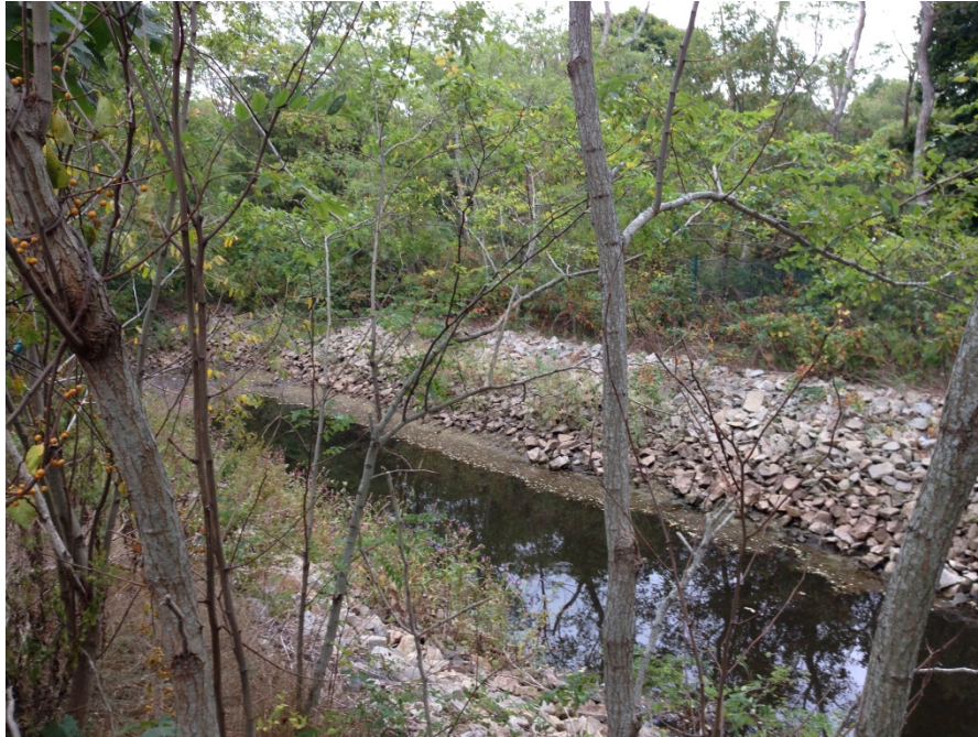
Photo 1. Infiltration basin adjacent to Route 28.
