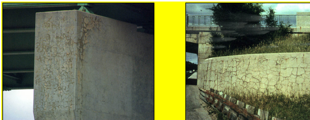
(a) Moderate ASR Cracking
