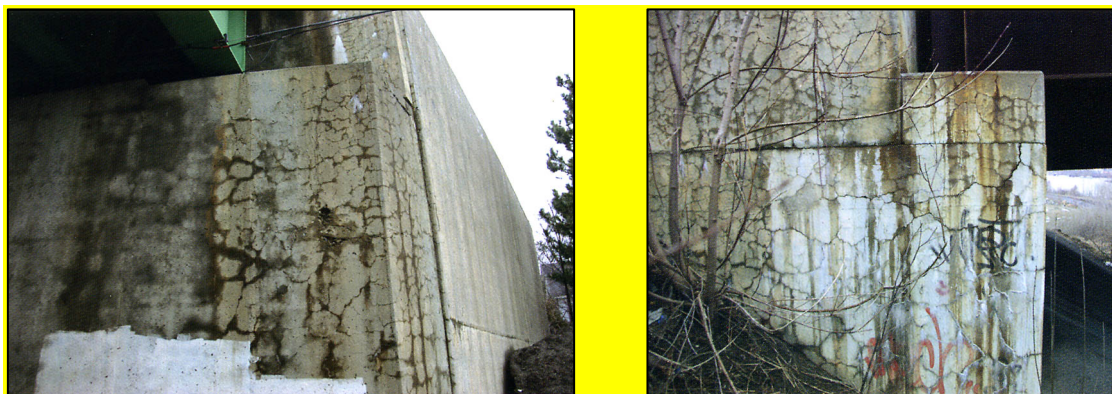
(c) Severe ASR Cracking
