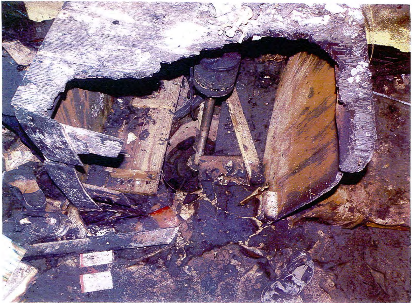
4(f) - 627 Pleasant Street, Winthrop – Sump pump in basement floor
