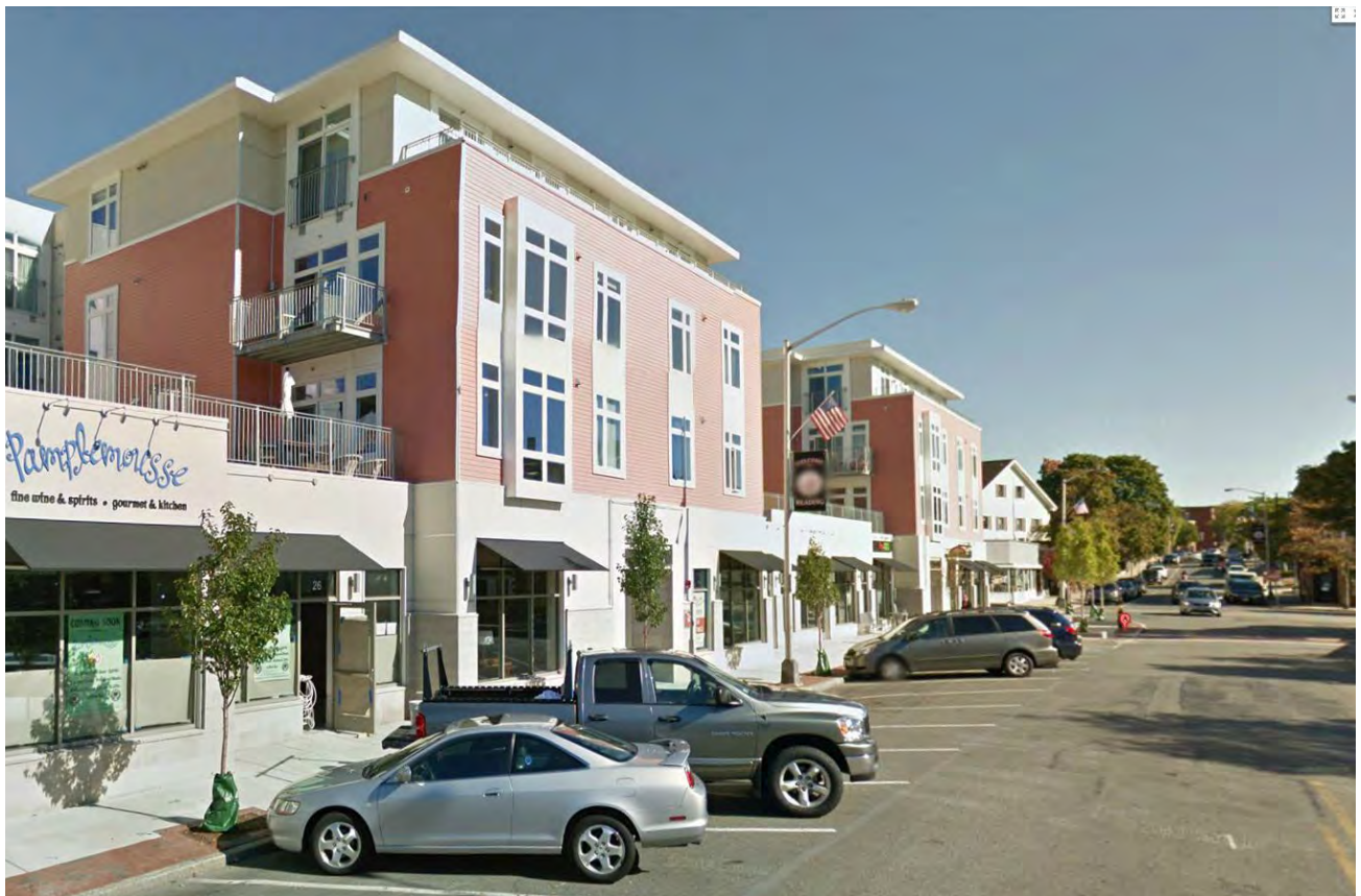
STREET VIEW OF COMPLETED 30 HAVEN STREET APARTMENTS
