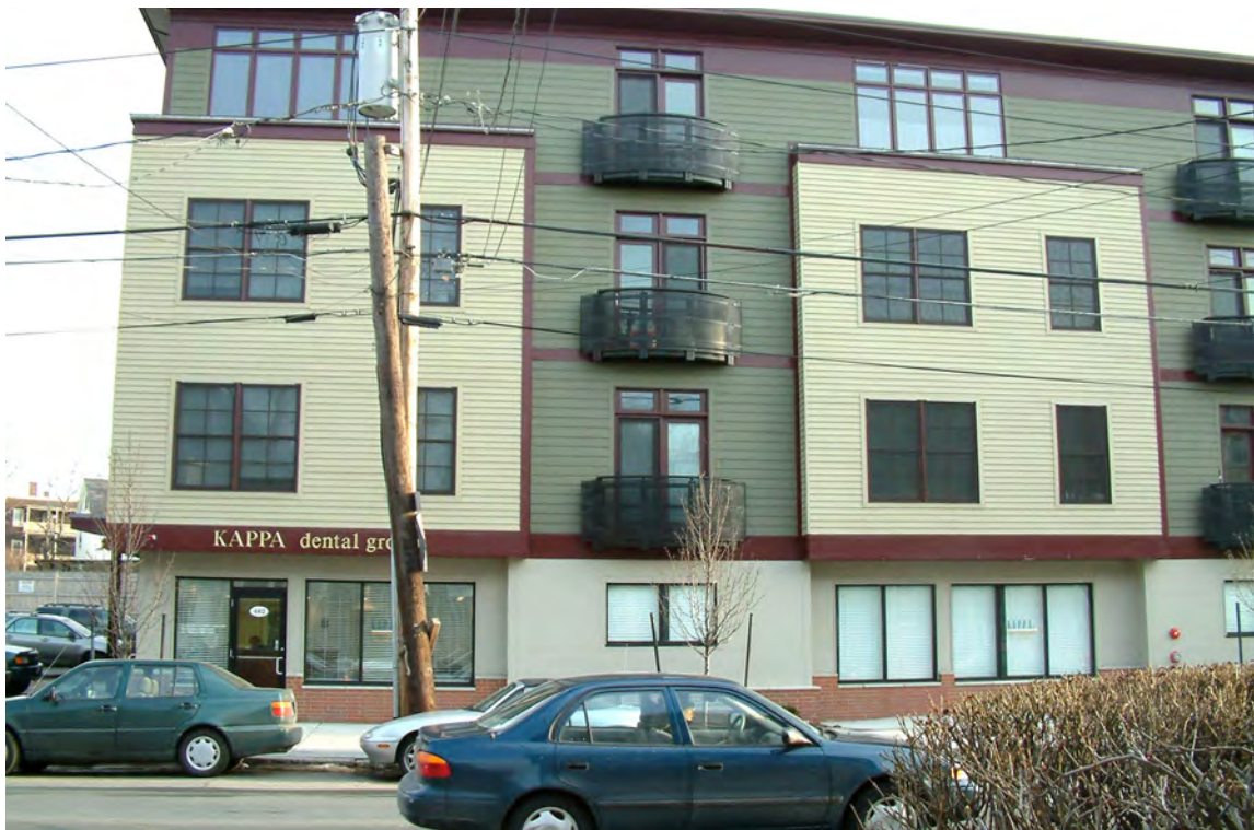
Mixed-Use Building, Cambridge, MA
