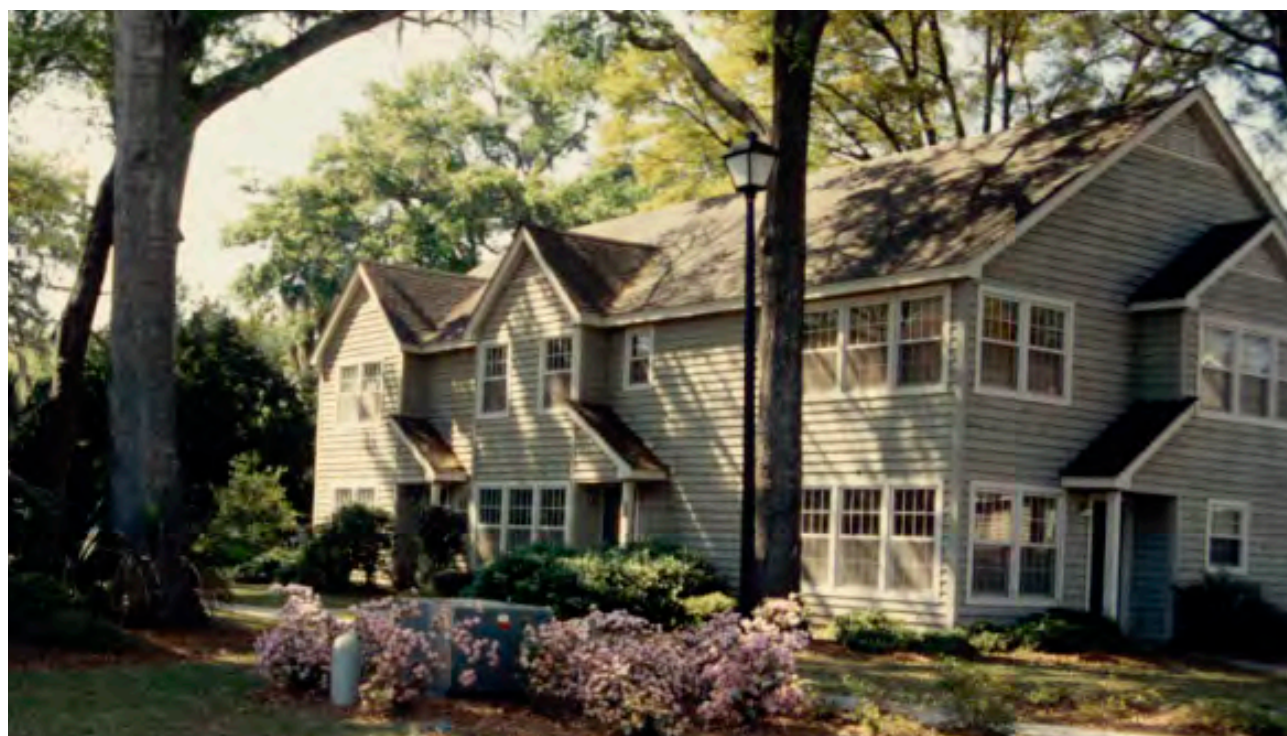
Single family massing and detailing can include as many as six apartments.
