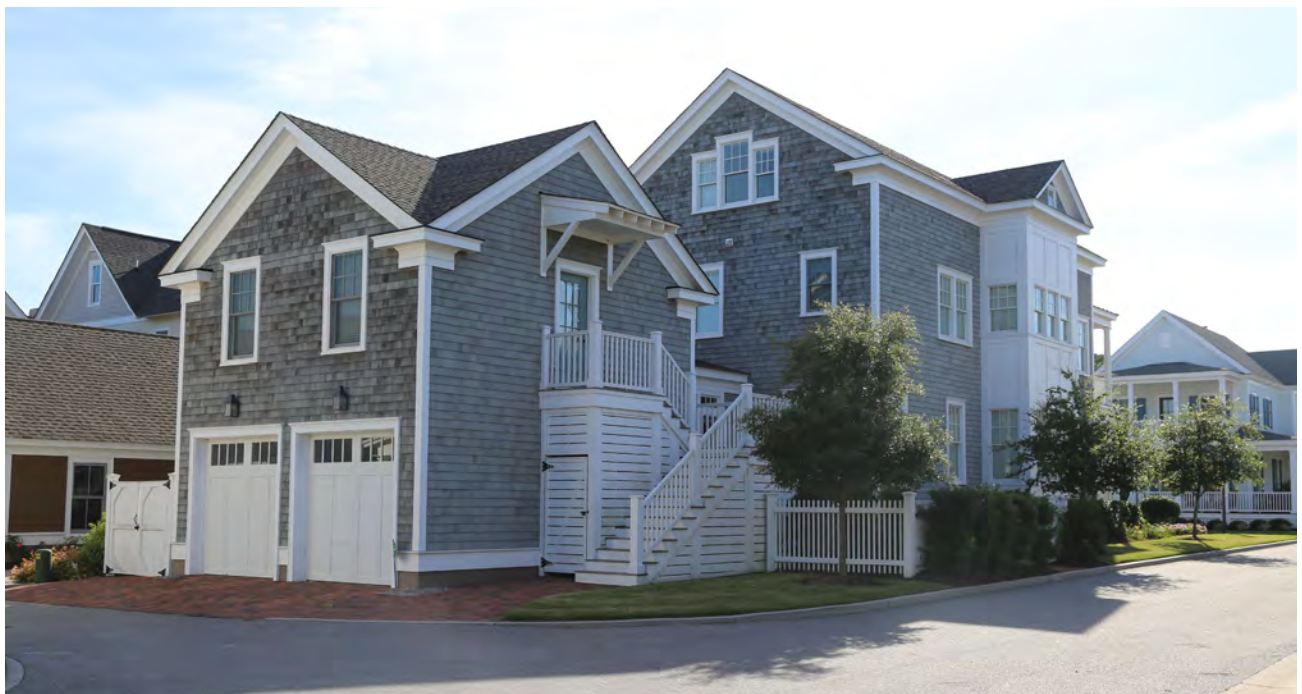
Three family: Two flat main house with accessory flat over garage, East Beach, VA
