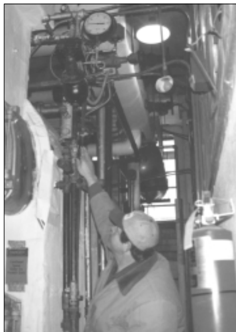
Inspecting building components is an important part of preventive maintenance.
