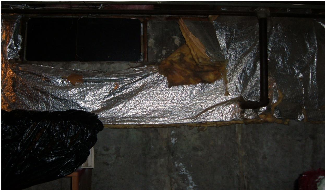
**200-1 Development, Normandy Road –Heating Duct Insulation Peeling from Basement Ceiling**
