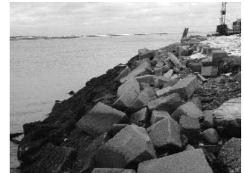
Riprap is commonly used to secure the shoreline where erosion is a problem.
