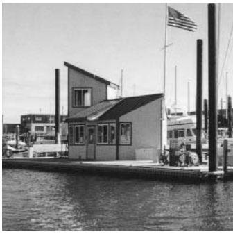
Fueling dock at Hewitt's Cove Marina.
