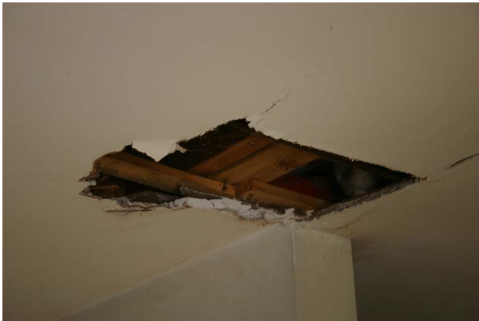
705-2 Development, 7 Chandler Way Kitchen – Ceiling Has a Large Hole That Needs Re-plastering
