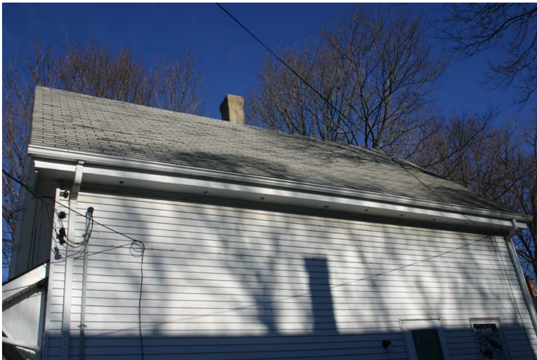
Scattered Sites 705-1 Development, 28 Barrows Street Roof in Need of Replacement
