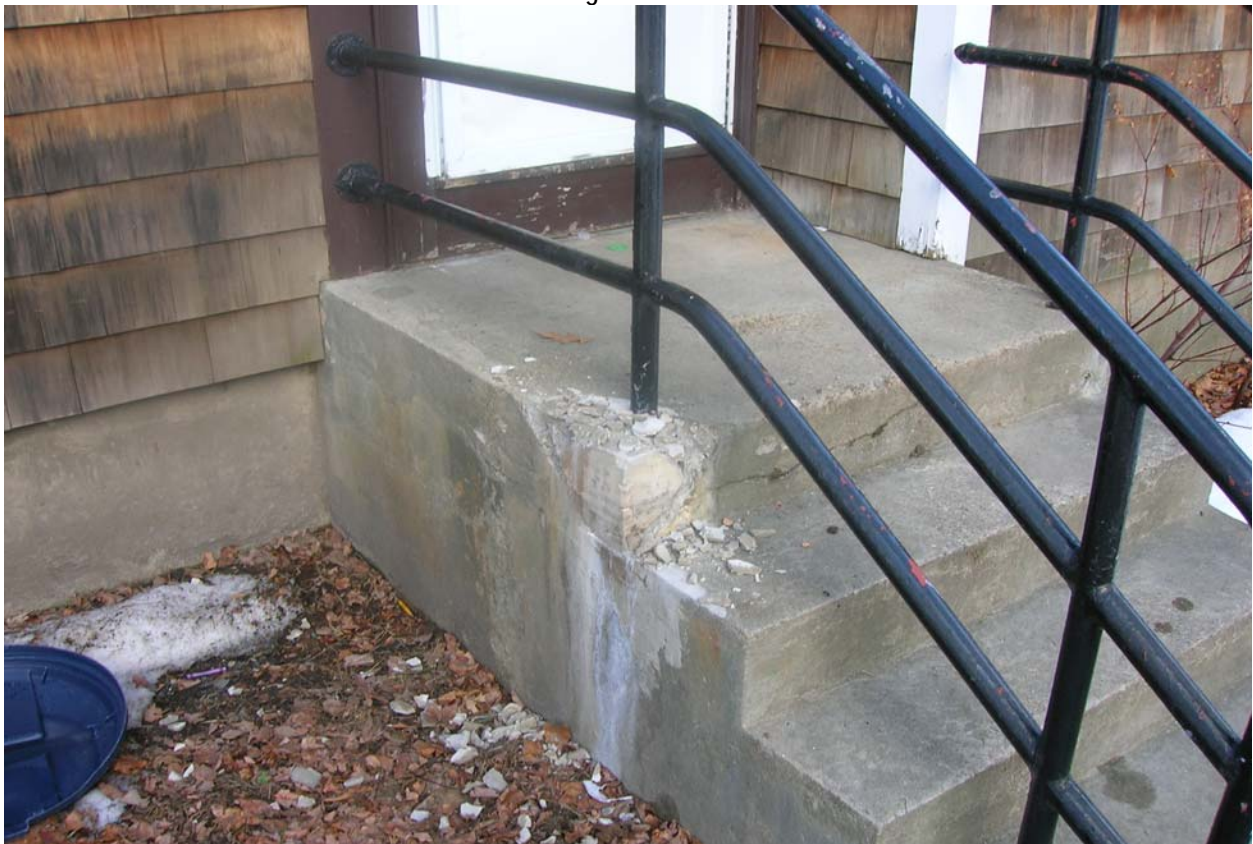
200-1 Development 112 Oakside Avenue Crumbling Concrete Stairs
