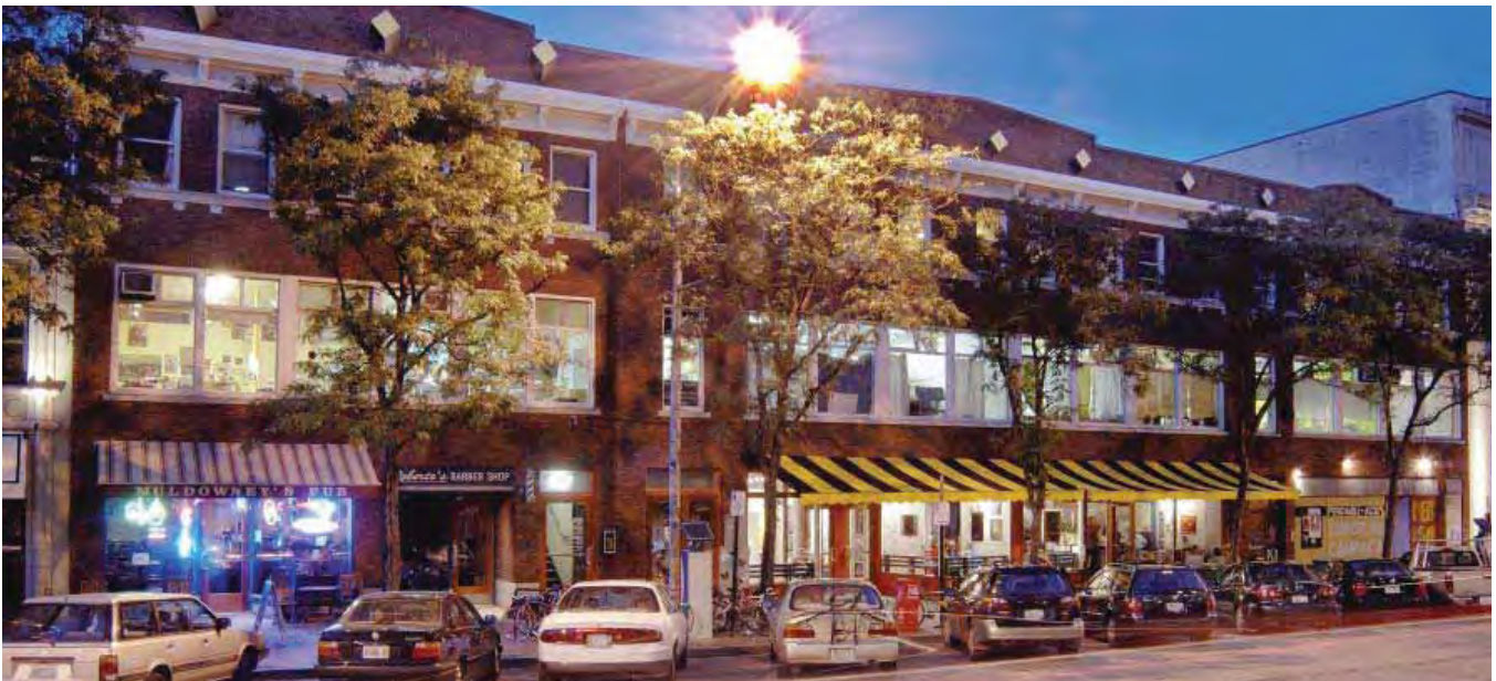
Location: Providence, RI Size: Five Buildings Client: AS220 (AS220 Exhibition Space , Perishable Theater) Trinity Repertory Company (Pell Chafee, Lederer Theater Complex, Administrative Offices) Cornish Associates (Packard Building, The Harkness Building)
