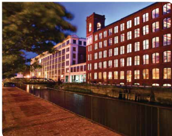
Washington Mills Building No. 1, Lawrence, MA. An award winning project done in collaboration with Durkee Brown Viveiros & Werenfels
