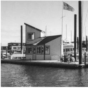
Fueling dock at Hewitt's Cove Marina.
