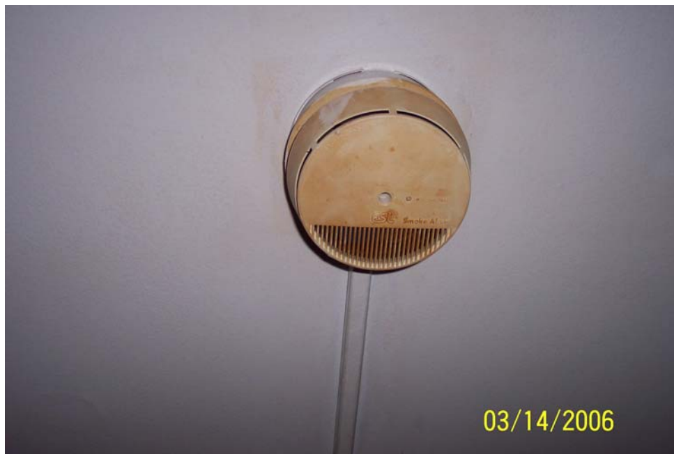
667-1 88A Forest St., #10 – Smoke Detectors Need Replacement
