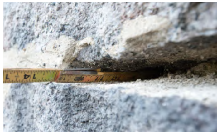
14.4: Open joint on east facade where the original lime mortar behind the 1900 cement pointing has been reduced to sand.
