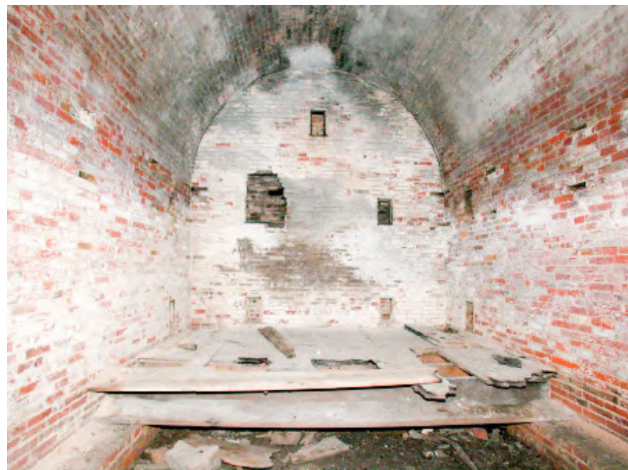
5.7: Current view of the interior of the Fort Pickering magazine. It is not known if it had wood lining the walls. The remnants of whitewash on the bricks suggests it did not. The rectangular openings are indirect vents.
