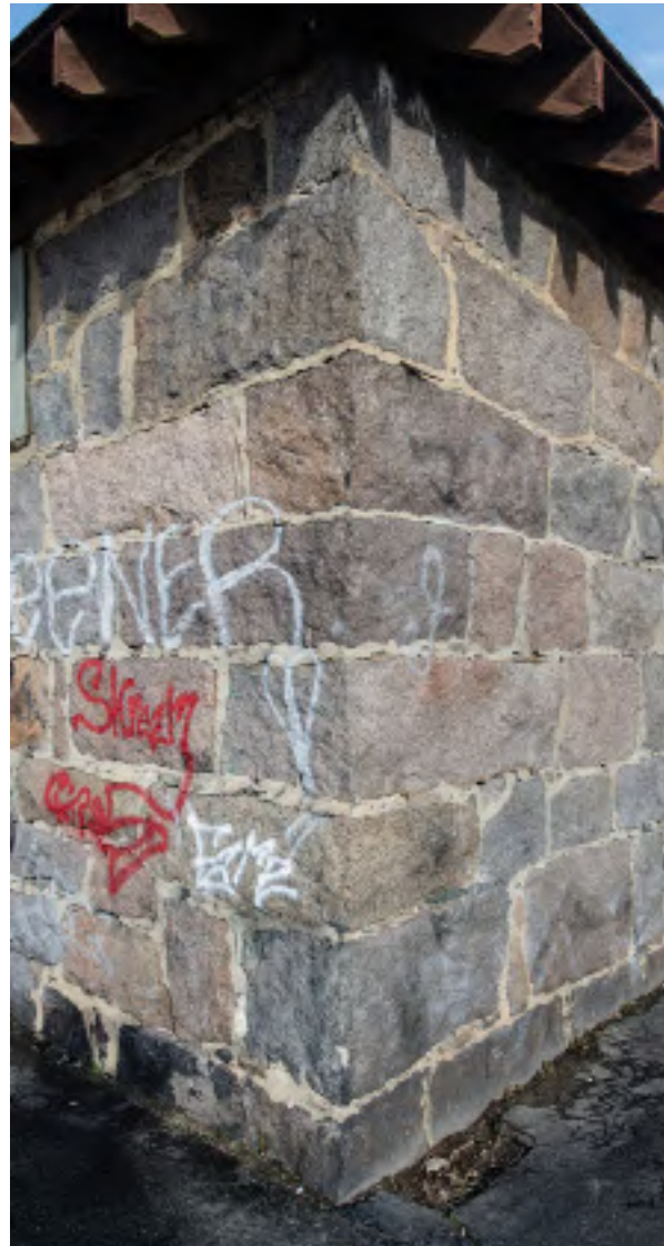
14.1: Southwest corner of magazine showing that 3'-4' long stones were alternated in each course to firmly tie the corner together.
