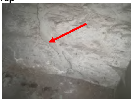
Photo 4: Crack in interior face of addition's west wall at south end. (Three close-up photos)
