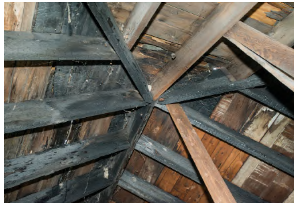
17.5: Detail of junction of main ridge with west hip. The sheathing and rafters of the west hip (upper center right corner) are obviously newer wood. The original rafters show surface char as do the few remaining boards of original sheathing.
