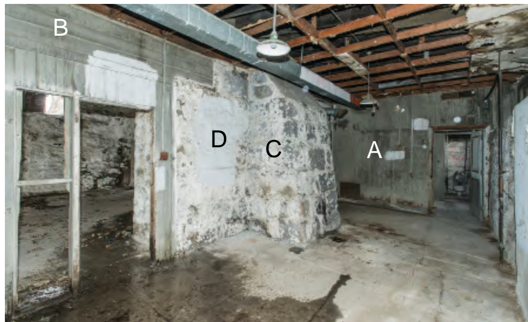
20.4: Overview looking east with the exterior face of the original 1818 north wall of the magazine on the left. The partition "A" was installed without the current door in 1918 to define the space beyond it for the storage of rental bathing suits and towels that was entered from the magazine. The boards at "B" were installed in 1918 to replace 1899 windows. The infill below "B" was built sometime after 1918 to fit the opening with a door. "C" marks the 1818 buttress that was partially rebuilt in 1899. The heating duct and lamps date to 1954. The fiberboard ceiling and its framing are likely 1954 or later. The cement floor dates to 1918. A sink was installed in 1918 below the plaster on the wall at "D".
