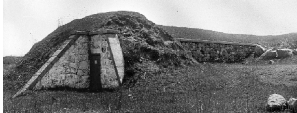
5.1: 19th century photograph of a powder magazine at Fort Pickering in Salem that is typical of magazines constructed within fortifications. It is partially below ground and covered with earth in order to make it more bombproof.
