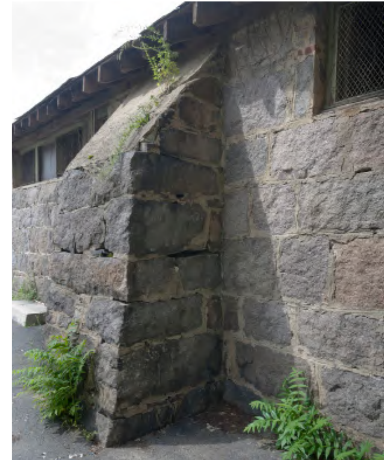
14.3: Overview of buttress at south facade showing substantial mortar defects with plants growing out of some joints. Some rebuilding of this buttress may be needed.
