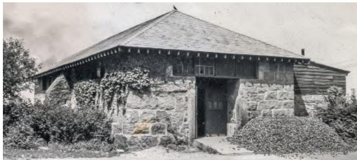
9.4: Photograph dated 1941 of the east end of the magazine showing several alterations made since 8.3 was taken in 1932. A concrete ramp has been added at the door, probably to facilitate moving items for storage into the building. The pile of gravel or debris to the right of the door suggests the building is now being used for maintenance purposes rather than as a bath house. A stack is now visible above the roof of the addition. Based on 3' x 3' x 4" concrete platform that is still present on the floor at this location inside the addition, the stack may have been to vent a stove to heat the addition for the maintenance staff.
