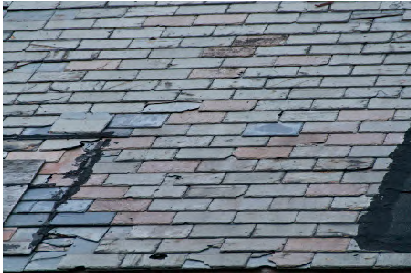
16.1: Section of the south pitch of the magazine roof showing the variegated color of the slates from grey-green to light tan. This is typical of the “sea green” slate specified in the 1918 drawings. They are a type also known as “weathering green” because they change color as they weather. They were less expensive than “unfading green” slates which do not change color and last substantially longer than weathering slates.
