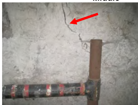
Photo 2: Diagonal Crack in interior face of main building's south wall at west end. (Three close-up photos)
