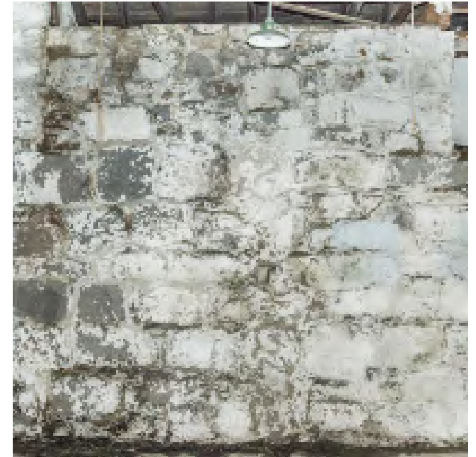
19.3: Detail of north wall (18.2 at the yellow dotted line) showing the smaller, irregular stones where the wall was rebuilt above the spring of the arch and where the central partition was removed.
