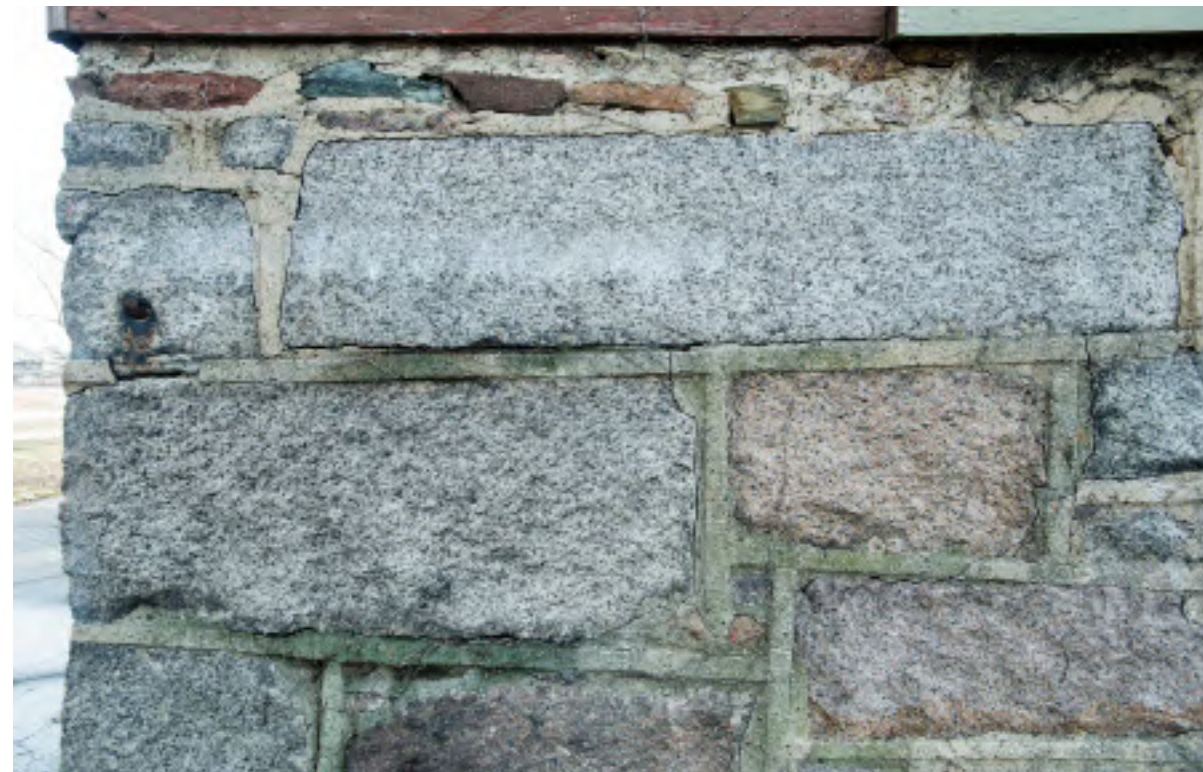
15.3: Detail at east end of north wall of 1899 addition showing the original mortar joints finished with a raised rectangular profile. Repointing on the addition should duplicate this profile. The small stones at the top are probably 1918 work to provide a level bed for the wood wall and windows.
