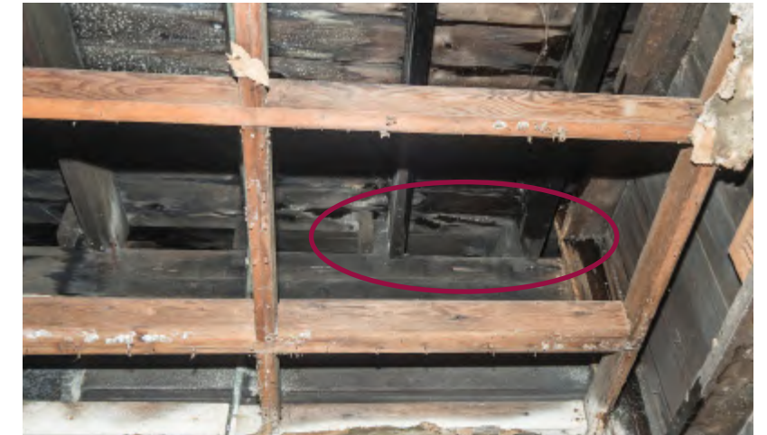
17.6: Interior of 1899 addition looking towards its junction with magazine north wall. The lower light colored framing was installed with the fiberboard ceiling. White spots on the ceiling are probably fungus from dampness.
