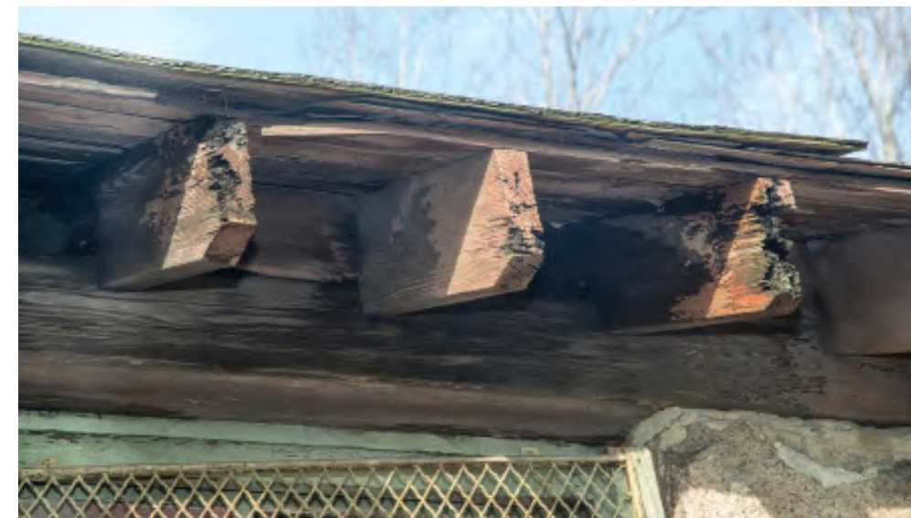
16.5: Detail of the roof edge at the south facade showing more typical rot in the rafter tails than in 16.4. At least 20% of the rafter tails show this level of deterioration due to uncontrolled drainage off the roof edge. In the 1899 construction a gutter was placed over the rafter tails, but was removed in the 1918 alterations. Exposed end grain is particularly vulnerable to deterioration when water drains over it.
