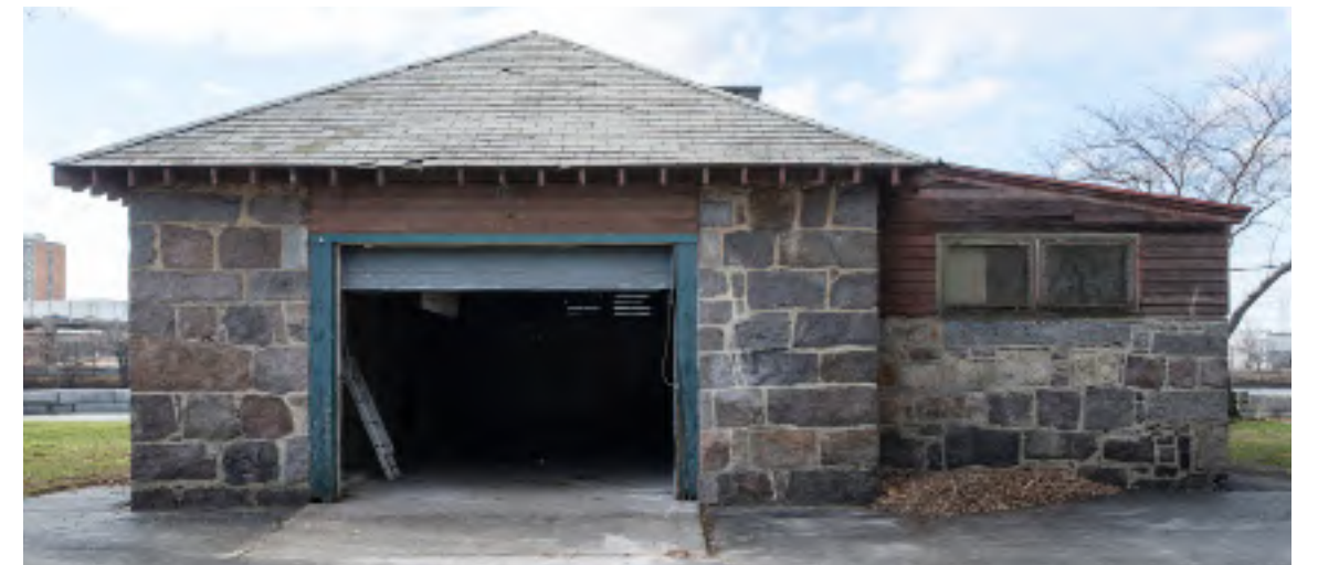
13.4: East elevation. The entry door was widened and the window above it removed and blocked in 1954. Windows in east end of addition were also added in 1954.
