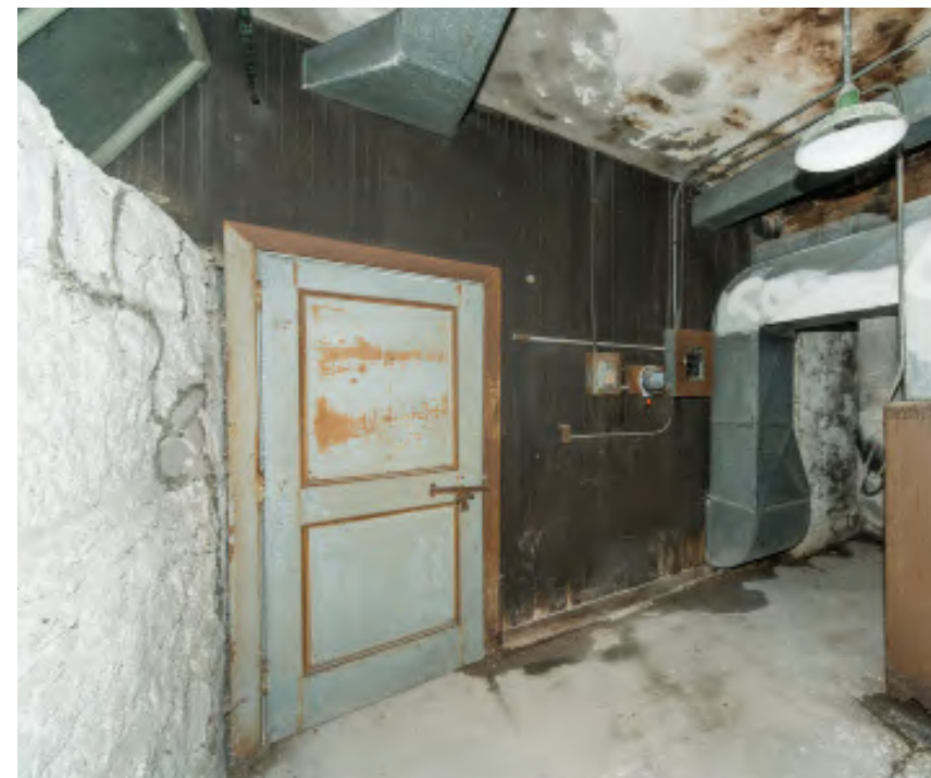
20.5: Current utility room at the east end of the 1899 addition, looking at the other side of the matched board wall marked "A" in 18.4. The kalemene (metal-clad) door was installed in 1954 when the current furnace and ductwork were installed.
