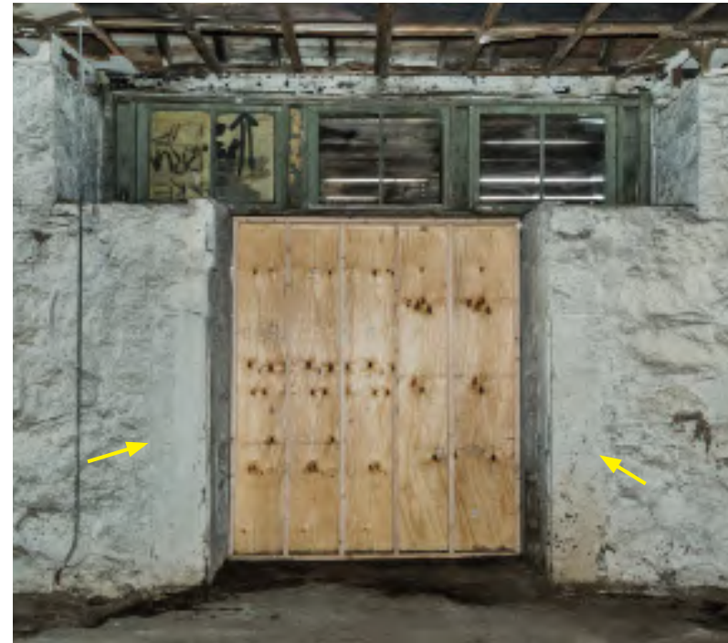
19.2: West end showing the modern infill of the door opening. The opening was widened to this width and height in 1918. The original granite jambs (arrows) were repositioned to their current location in 1918. The original jamb stones are also present on the exterior side. That a set of jamb stones was placed on both the exterior and interior indicates there were probably inner and outer doors when the building was used as a powder magazine.
