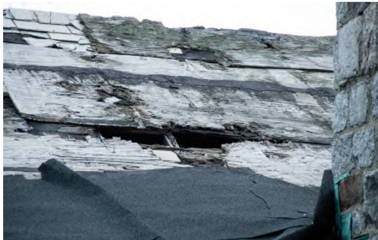
16.3: Detail of the south pitch of the magazine roof above the chimney showing that not only is the slate gone, but the plywood put on to patch the roof and sheathing below it is now severely rotted. The copper flashing for the chimney is also in poor condition and needs to be replaced if the chimney is retained (the chimney was added in 1954).
