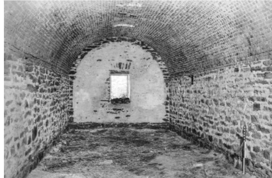
5.2: Photograph of interior of powder magazine at the US arsenal in Pikesville, Maryland. A note on the HABS drawings of the magazine says "The building was formerly lined with wood sidewalls, ceiling and floor. All fastenings were counter-sunk and plugged to avoid a possible spark. The pintles are of bronze." The magazine may be as early as 1816. It was surrounded by a wall as shown in the sections below.
