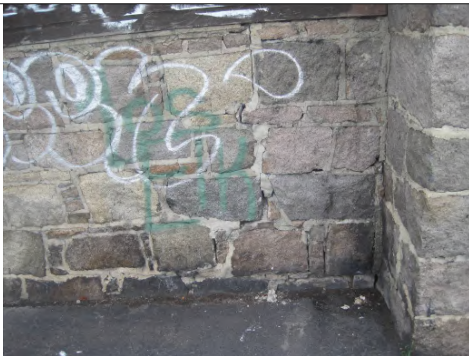
Photo 11: Typical exterior wall stone joint deterioration (west side of building)
