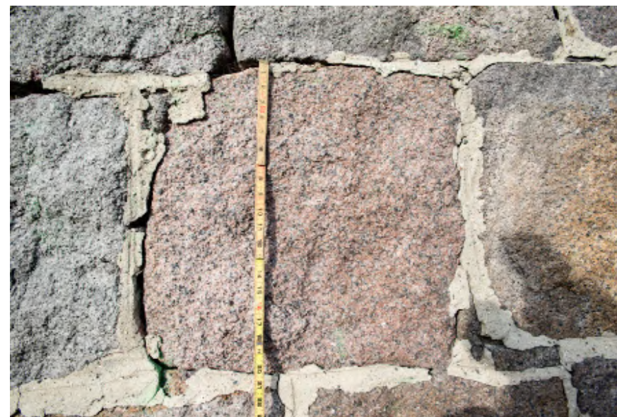
14.5: Detail of south facade showing the typical size of the stones along with the poor condition of the 1900 pointing. Despite the poor condition of the mortar, the stones show little evidence of movement except for the one crack noted in the engineer's report.
