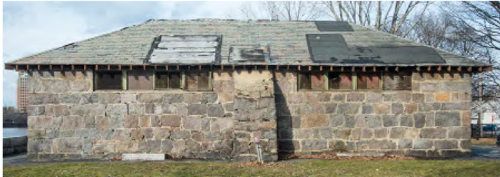
13.1: South elevation. The stone is laid in regular horizontal courses. Most stones have been dressed to roughly rectangular shapes. There is a considerable range in the color of the stones, which is typical of Quincy/Braintree granite quarried prior to c. 1825. There are numerous large patches in the slate roof.
