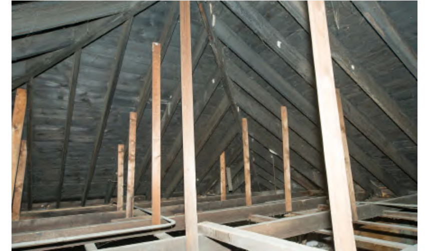
17.3: Interior of east hip at junction with south pitch (right). The rafters and sheathing in this section are mostly in serviceable condition and retain their original dark brown stain finish.
