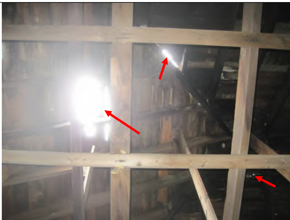
Photo 13: Roof damage from interior
