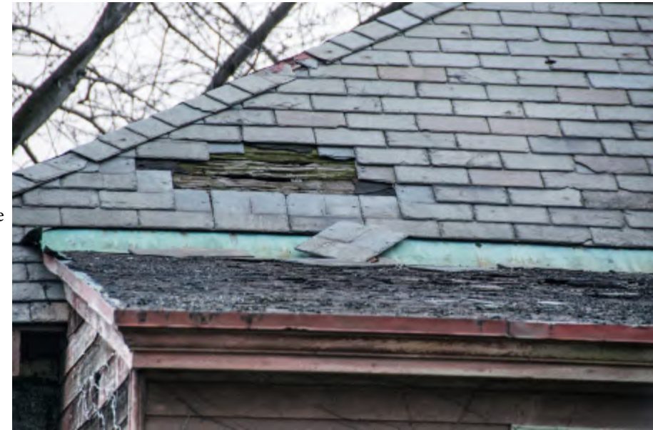
16.2: Section of the north pitch of the slate on the magazine, and the tar and gravel roof on the 1899 addition with a copper flashing apron between the two. Although most of the slates appear sound at this end, the sheathing boards where the slates are missing have rotted clear through. The tar and gravel roof is of unknown age (perhaps 1954) and is assumed to be well past its service life.
