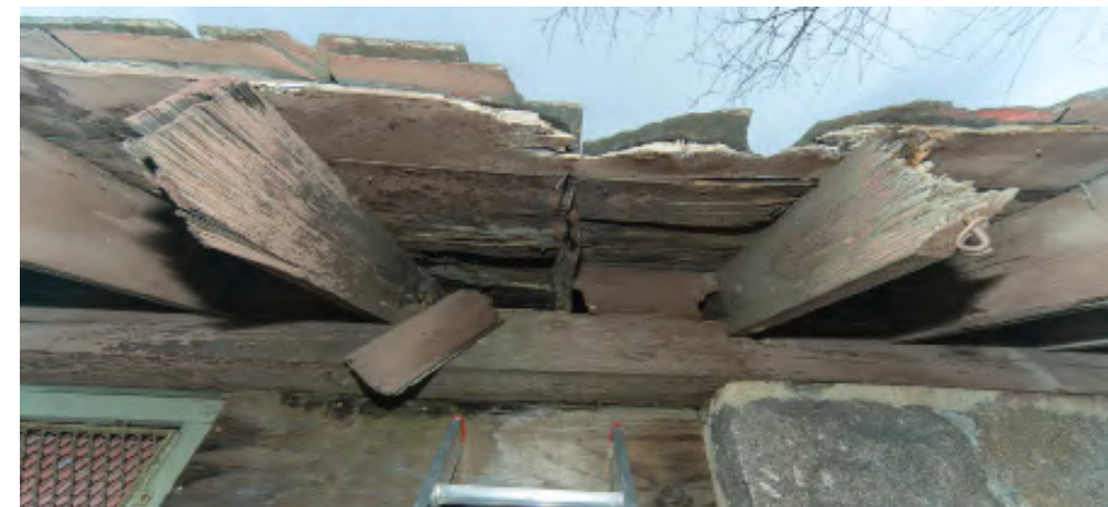
16.4: Detail of the roof edge at the south facade where the projecting rafter tails and roof sheathing are severely rotted due to uncontrolled drainage off the roof edge and broken slates. This is the most severe damage observed at the rafter tails, but many have minor damage as shown in 14.5 below.
