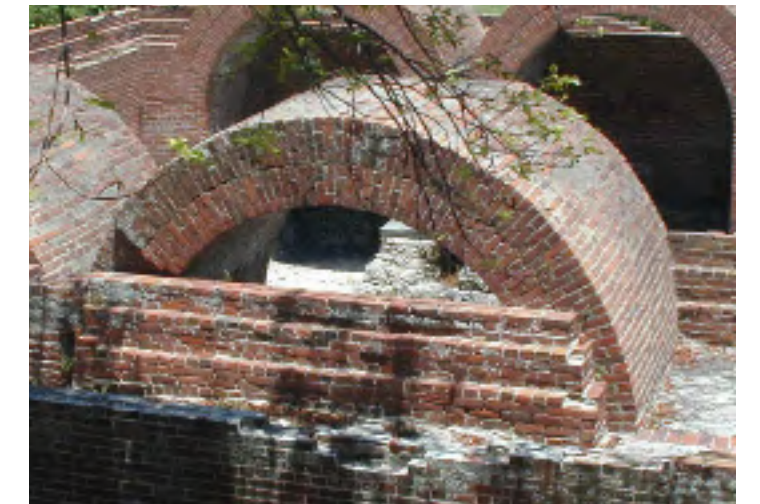
4.5: Ruins of fort at an unknown location showing the construction of a brick semi-circular arch similar to the arch in the Captain's Island Magazine. In this example the arch is 24" thick rather than 16".
