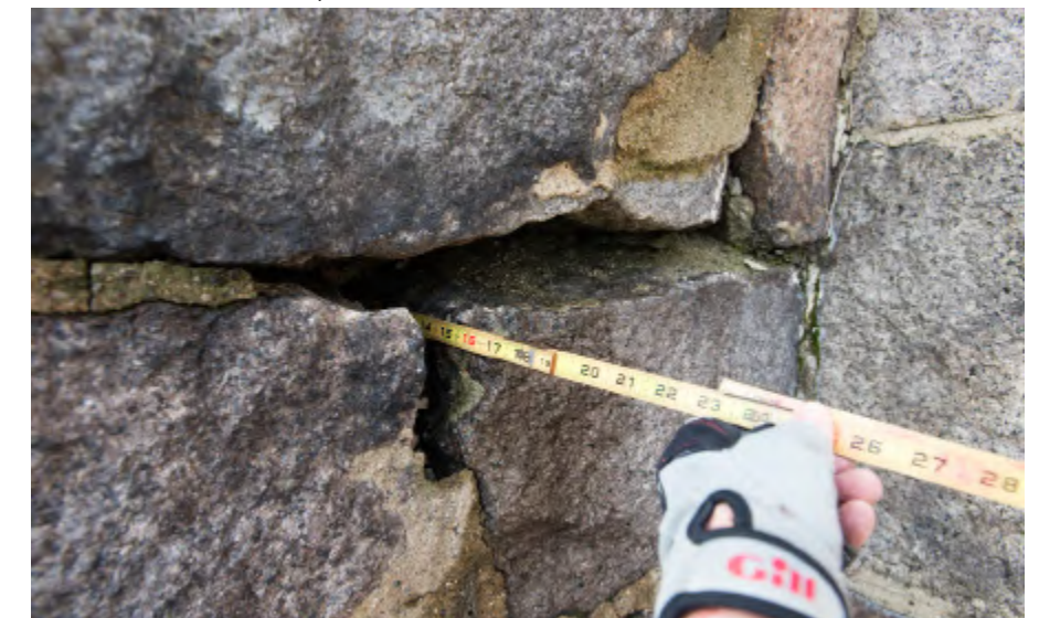
14.6: Detail of severely defective joint in buttress that is void of mortar 16" into the joint. The interior mortar may be very deteriorated. Rebuilding the buttress using the existing stones and coursing may prove necessary.
