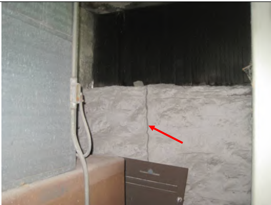
Photo 3: Crack in interior face of addition's west wall at south end.
