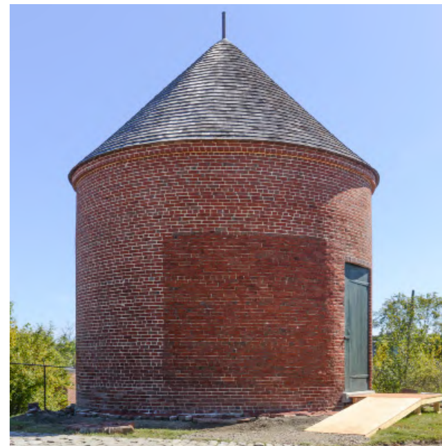
5.8: Newburyport Powder House. It is 18' in diameter and is typical of the structures built by towns for the local militia and powder merchants.
