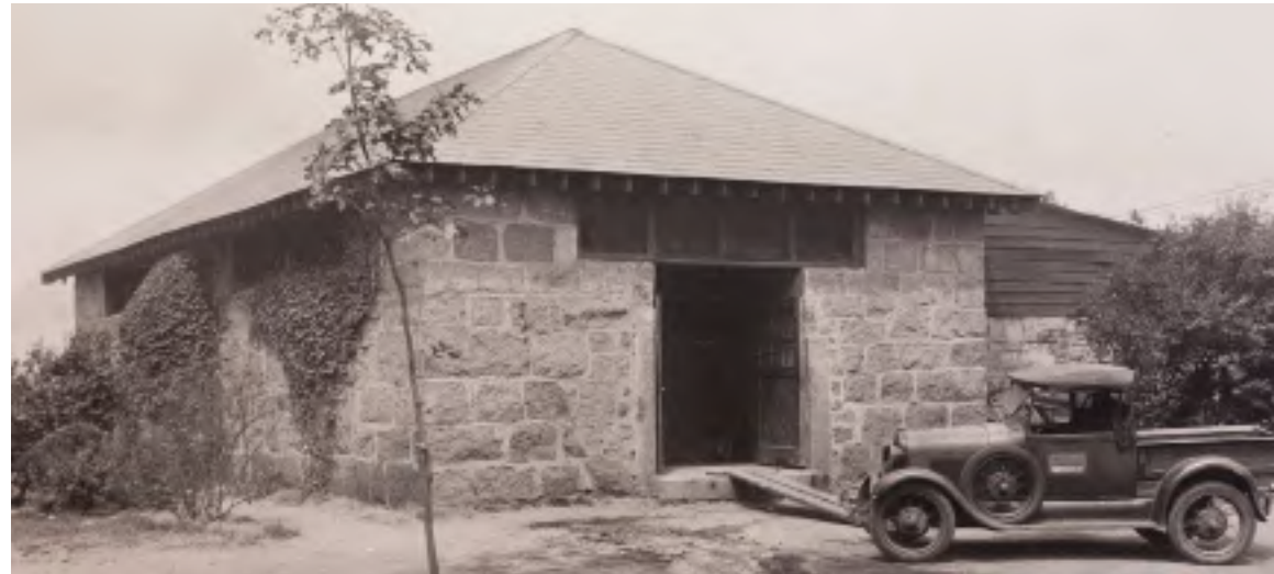
9.1: Photograph taken in the 1930s of the east end of the magazine showing the alterations made to the exterior in the 1918 renovation. The entrance has been widened to 7' and raised to the underside of the windows, the north addition has been closed in above the stone work, the wood shingle roof has been replaced with slate, and the gutters and downspouts removed.
