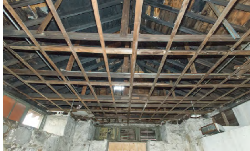
17.1: Overview of magazine ceiling showing the strapping for the fiberboard ceiling and the 2"x 6" tie beams with the roof rafters and sheathing above. The ceiling was probably installed sometime after 1954, and the tie beams are likely from the 1930s or 40s (char on some indicate they predate the c. 1950 roof fire). As originally constructed in 1899 the space was open to the rafters and sheathing which were stained dark brown. The roof space remained open in the 1918 renovation.
