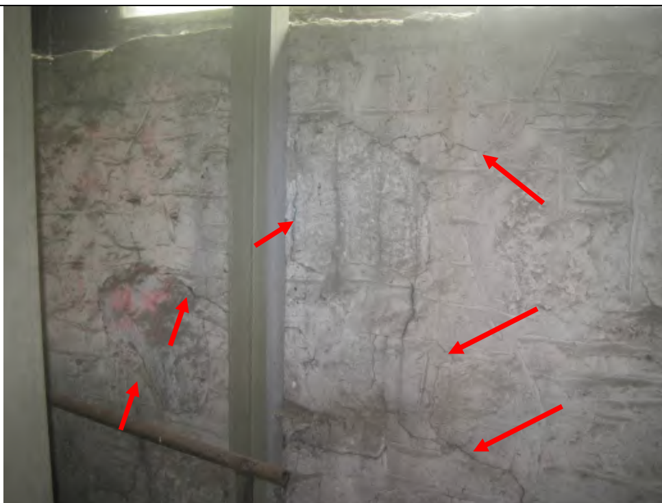
Photo 5: Spider cracking in the mortar joints at the interior face at the west end of the addition's north wall.
