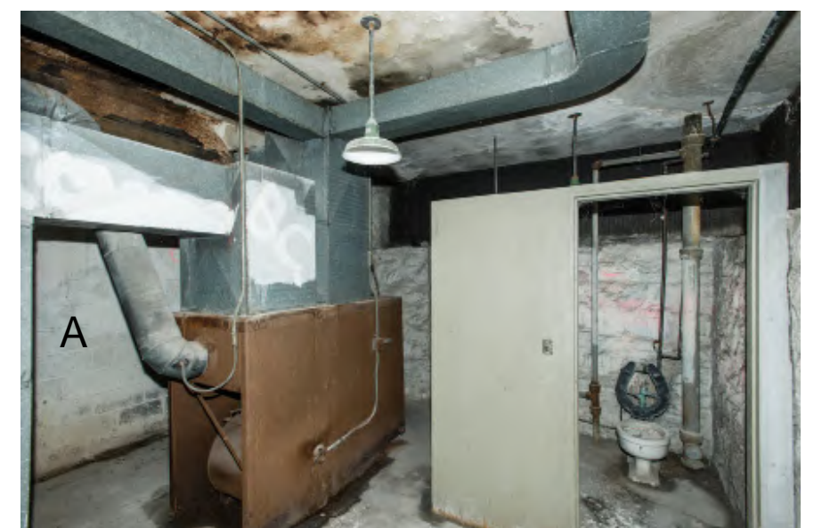
20.6: Current utility room looking toward the east end wall of the 1899 addition. The partition around the toilet was installed in 1954 along with the furnace and the plaster ceiling. The cement block wall at "A" was also installed in 1954 to infill the opening cut in 1918 in the north wall of the magazine to separate the utility room from the magazine space. As the furnace is over 50 years old, it is obsolete and should be removed along with its duct work. The plumbing and electrical systems also date to 1954. They have probably been damaged by the chronic dampness in the building. They are considered obsolete and should be completely removed. The design and installation of new mechanical and electrical systems should be based on the needs of the eventual reuse of the building.
