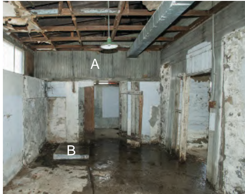
20.1: Overview looking east at partition installed in 1918 to separate the shower room. The matched boarding at "A" was added when the room was converted to an office, perhaps as early as 1940. The entry to the room was made narrower and a door added at that time. The cement platform at "B" was added after the urinal at this location was removed, probably c. 1940, to set a heating stove on.
