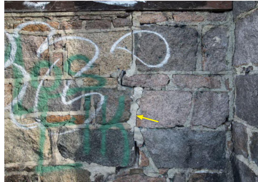
15.2: Detail of west wall of 1899 addition showing vertical crack through mortar joints (arrow) that corresponds to the edge of the masonry installed in 1918 to fill in the 1899 entry to the open yard. The color of the mortar in the 1918 joints to the right of the crack is slightly greyer than the 1899 mortar to the left of the crack. The crack extends clear through the 2' thick wall. Most of the mortar joints have hairline cracks at the their junction with the stone, and in some places the mortar has fallen out.
