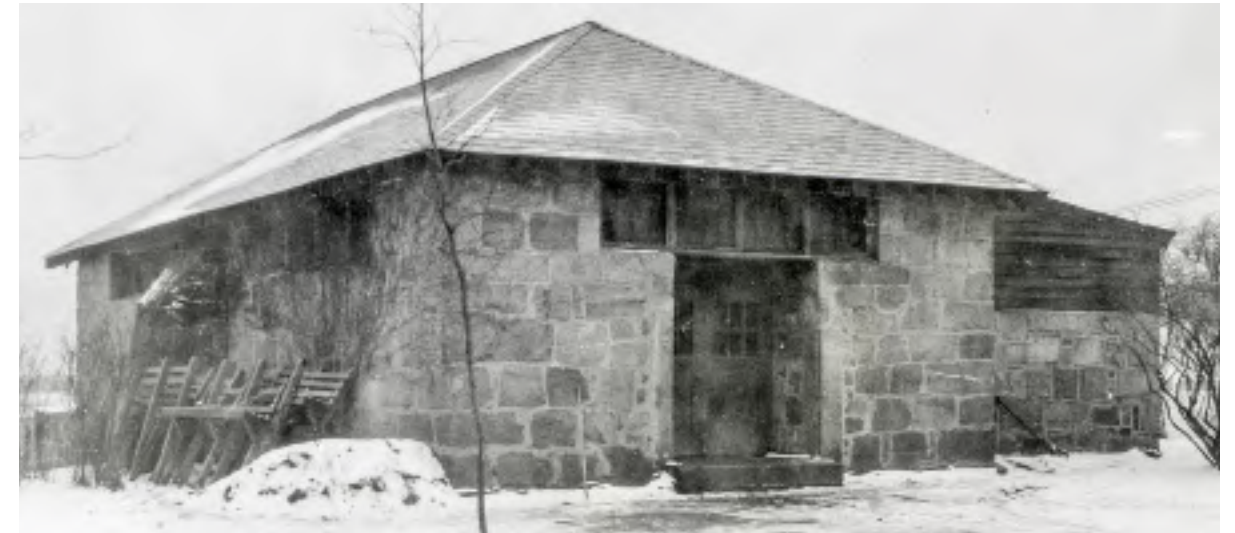
9.3: Photograph taken in the 1932 of the east end of the magazine showing the alterations made to the exterior in the 1918 renovation. Note that the bottom course of stone is fully exposed and there is a step to get up to the level of the interior concrete floor. The number of courses of the slate roof can be counted for comparison with the number of courses in the 1899 wood shingle roof in photo 8.6. Based on the extent of ivy growth at the corner, this photo appears to be a few years later than 9.1.
