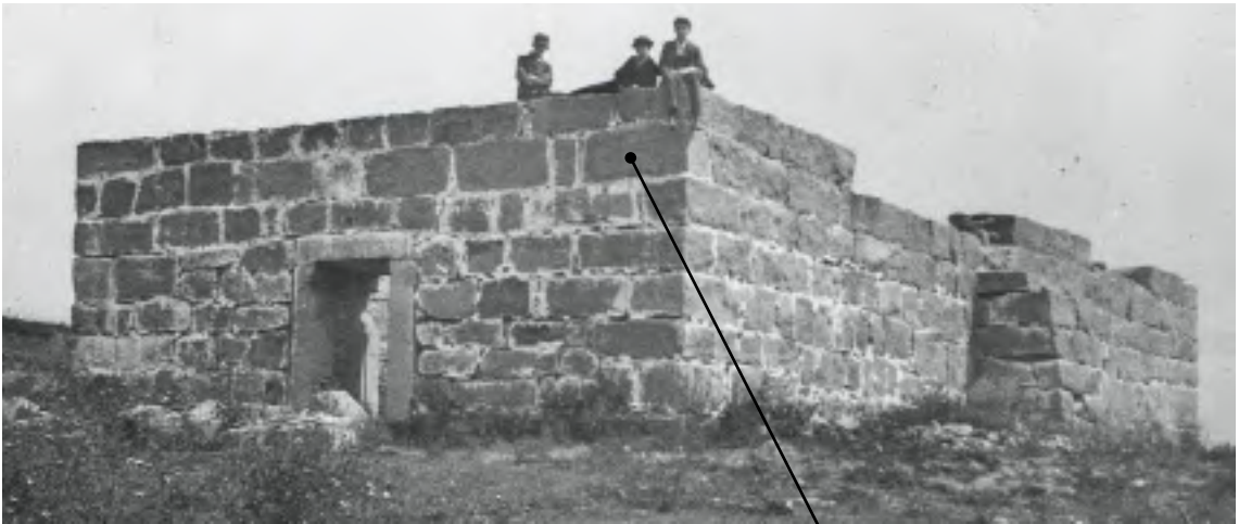
6.2 (above): Photograph of the west end and south side of the magazine from the 1890s showing its condition prior to being renovated in 1899 as a bathhouse. The slate roof, brick arch, and all doors are gone. The lower 8 courses (i.e., 11') of granite and the door openings remain intact, although portions of the eighth course are missing. The small chinking stones set in the joints also remain intact and are visible in this photograph. The top of the buttress is missing. There is no evidence of openings for ventilation (usually narrow slits) or windows in the remaining wall.
