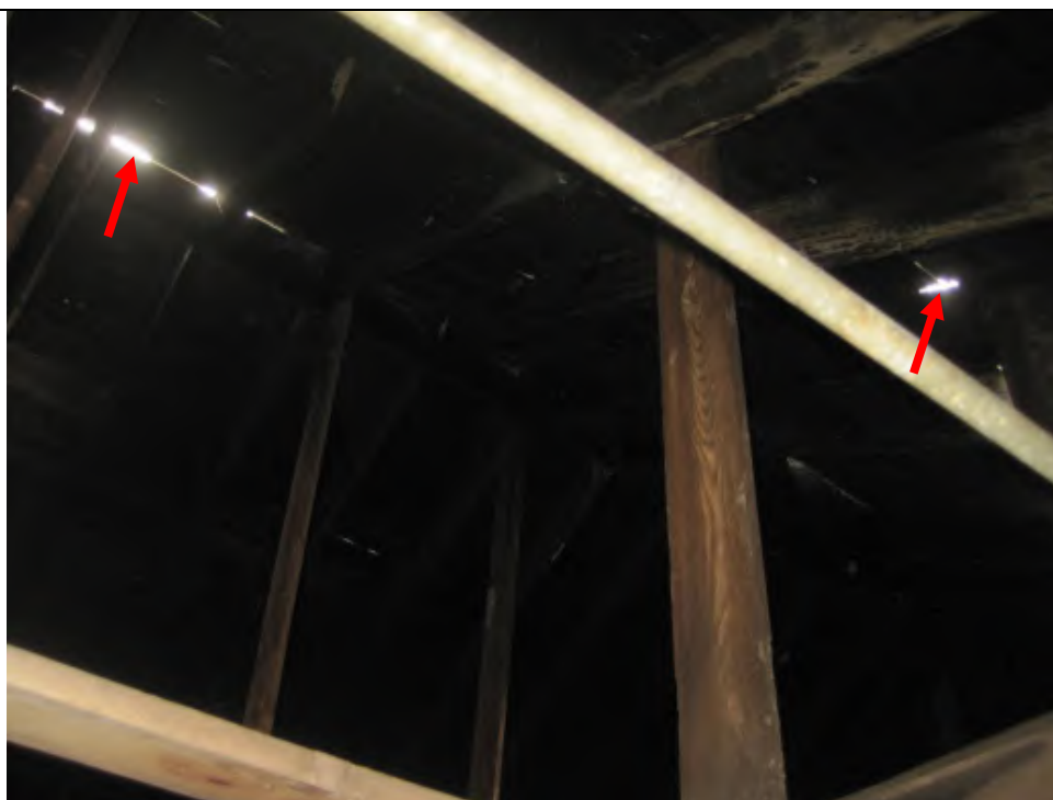
Photo 14: Roof damage from interior
