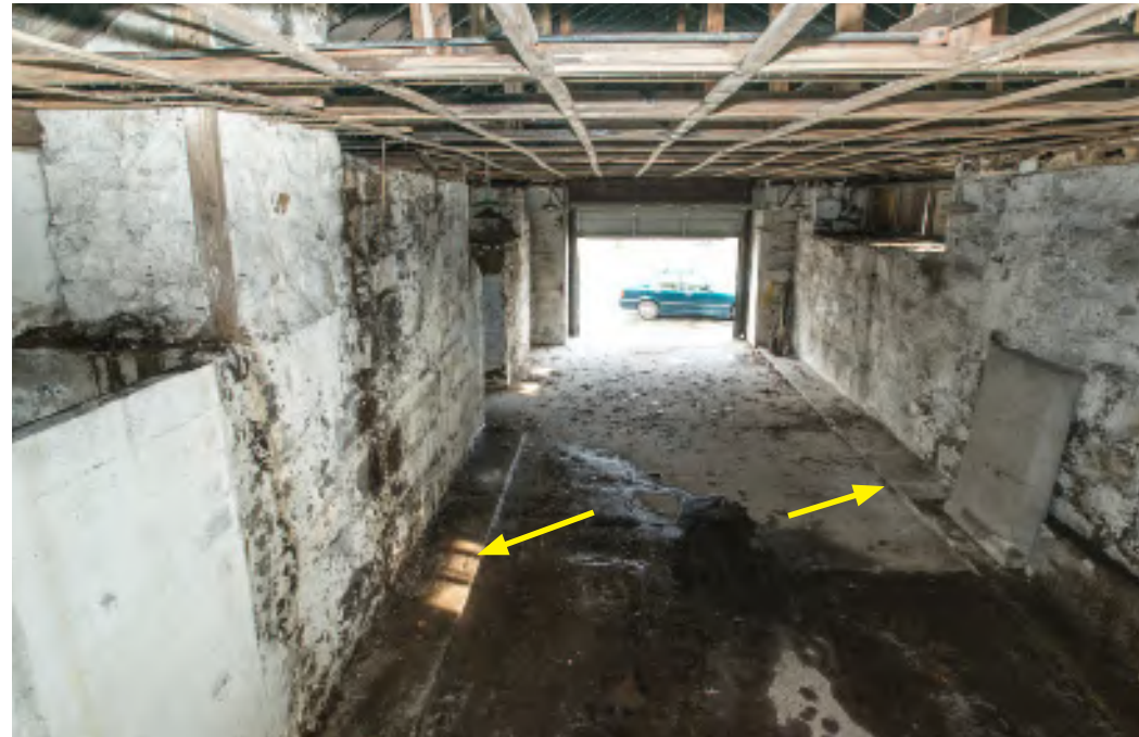
19.1: Overview of magazine interior looking towards east end entry. South wall is on the right. Yellow arrows point to raised platforms in the concrete floor that provided a base to raise the lockers above the floor. The concrete floor was installed in 1918. The previous floor was probably wood.
