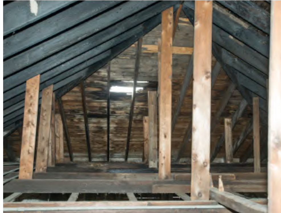
17.2: Interior of west pitch where rafters and sheathing were all replaced in 1954 due to fire damage. The vertical 1 x 6 struts were likely installed in 1954 or later as some are located on the section replaced in 1954. They were probably installed to support the framing for the fiberboard ceiling (i.e., tie beams and furring).
