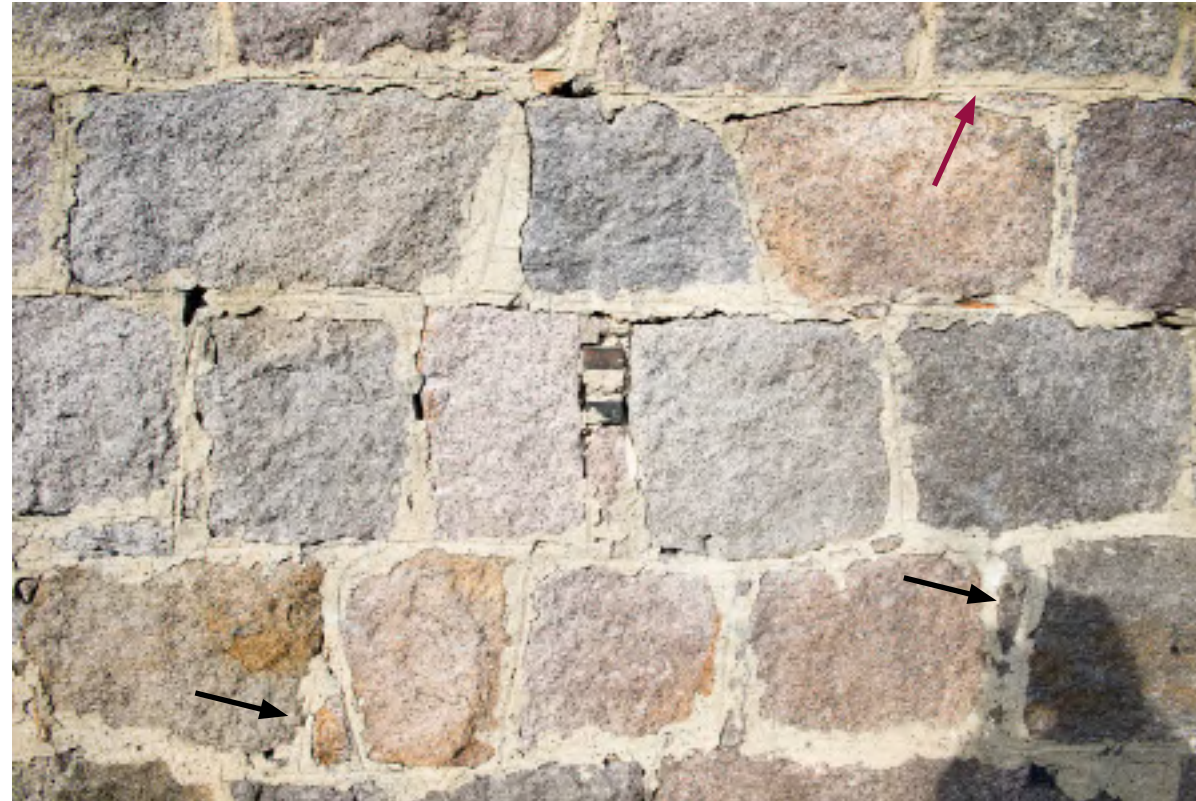
14.2: Detail of south facade showing the range of color of the granite includes pink and brownish stones as well as neutral grey. This is typical of Quincy granite quarried in the 18th and early 19th centuries before the large commercial quarries started c. 1825. Note the use of chinking with small stones to fill the wider joints between stones (black arrows). Much of this is original and should be retained. The pointing is probably from 1900 and now has numerous voids and cracks. The joints were tooled with a concave line along their centers to try to make them look neater (red arrow).
