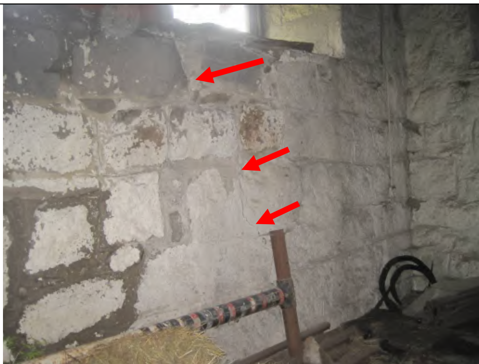
Photo 1: Diagonal Crack in interior face of main building's south wall at west end.
