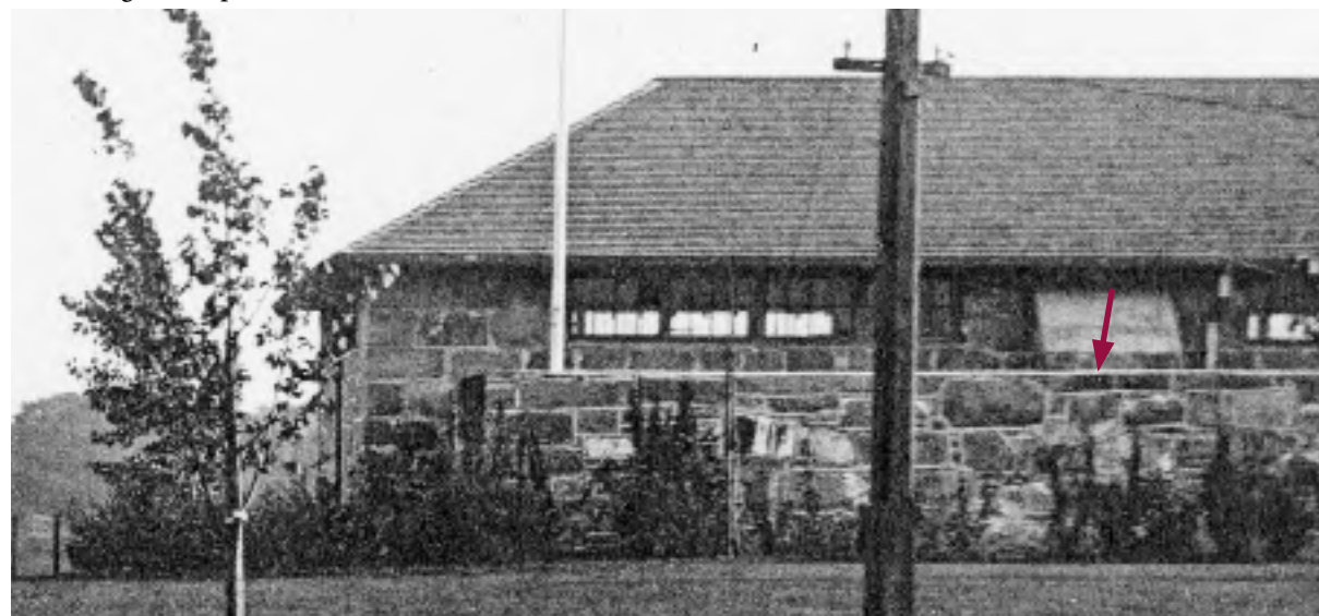
8.6: Detail of photograph from Cambridge Parks Dept. Annual Report of 1901 showing the east end of magazine and the 1899 north addition (arrow) that enclosed an open yard. The 8 light sash in the magazine are clearly visible, as is the gutter with a downspout on the right side of the photo. The large number of courses in the roof indicate it is wood shingles rather than slate. The white post at the left side of the addition is a flag pole.
