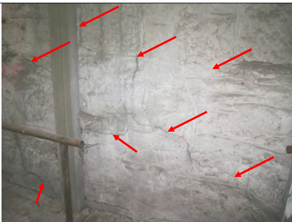
Photo 6: Spider cracking in the mortar joints at the interior face at the west end of the addition's north wall.
