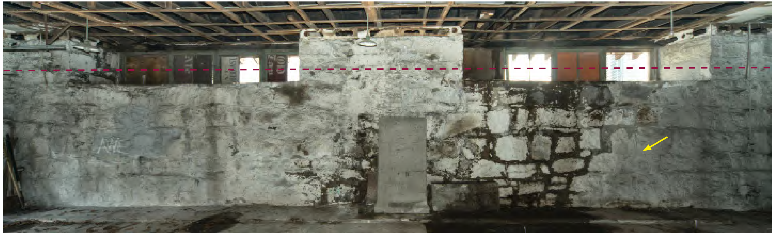
18.1: Overview of south wall in magazine. Dark joints are sloppily repointed joints using an inappropriately dark colored mortar. The crack discussed in the engineers's report is barely visible and is marked with the arrow (see 19.6 for a close up). The red line marks the approximate position for the spring of the 16" thick brick arch in the magazine as built in 1818. The stones above this line would have been missing for the 16" depth of the arch and would have been rebuilt in 1899.
