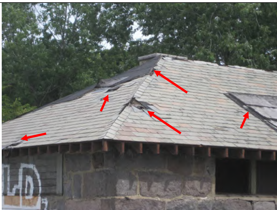
Photo 12: Roof damage from exterior
