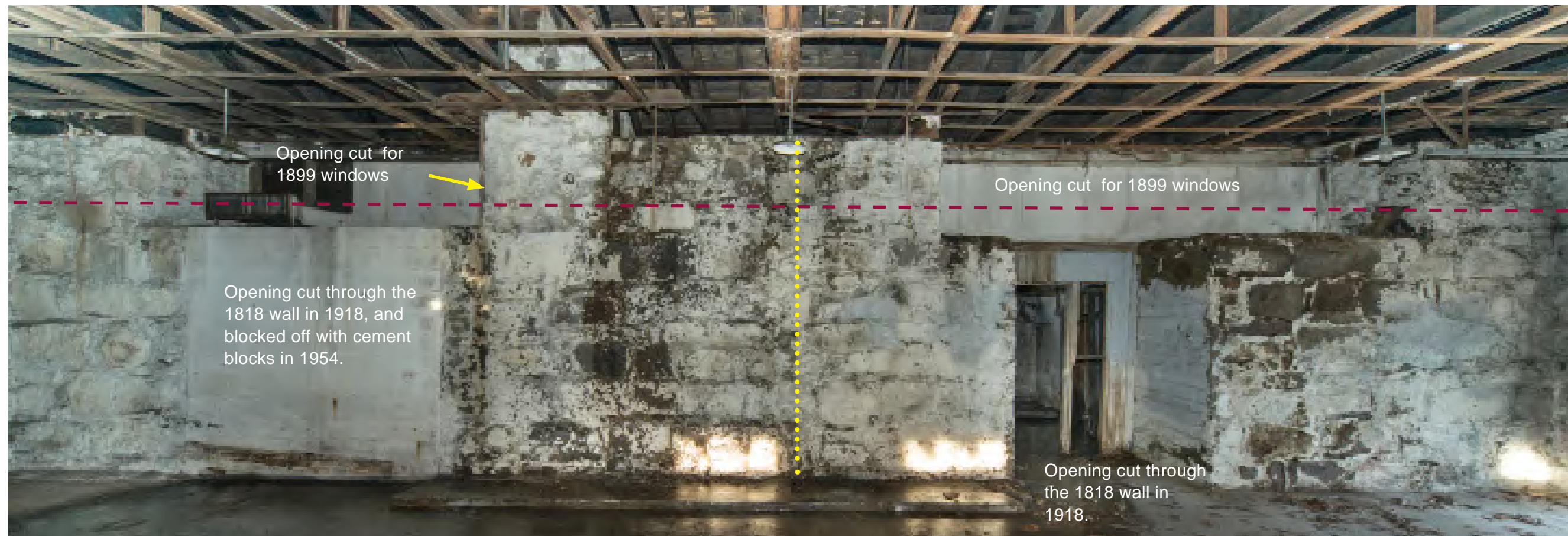
18.2: Overview of north wall in the magazine. The red line marks the approximate position for the spring of the 16" thick brick arch in the magazine as built in 1818. The stones above this line would have been missing for the 16" depth of the arch and would have been rebuilt in 1899. Most of the stones above this line are relatively small and irregular. The stones along the yellow dotted lines are also small and irregular. This indicates where the original interior partition was located and removed in 1899. The yellow arrow marks the base of the chimney added in 1954.
