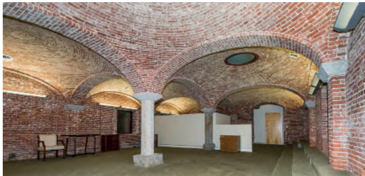
4.7: Interior of the Chelsea magazine showing the sophisticated shallow brick domes springing from segmental brick arches that Parris used to form the ceiling of the magazine. It is thought that he used a similar system in the 1817 Watertown magazine.
