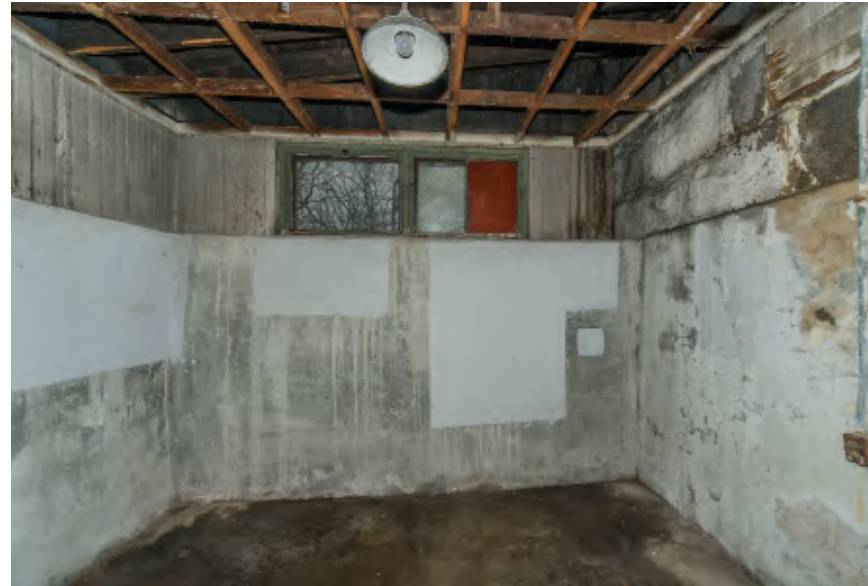
20.2: The cement plaster was placed over the stone in 1918 to make this a shower room. The room was later made into an office, perhaps c. 1940. The windows were added in 1954.
