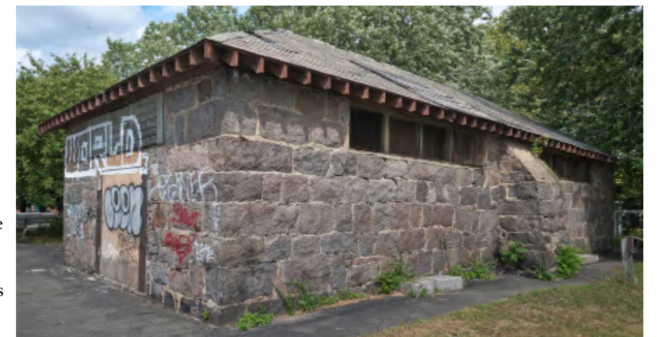
13.4: East elevation. The entry door was widened and the window above it removed and blocked in 1954. Windows in east end of addition were also added in 1954.
