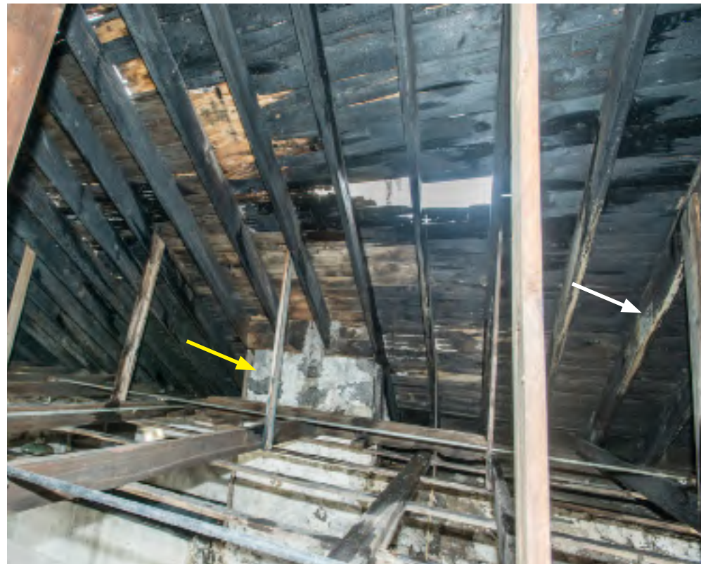
17.4: Interior of north pitch above chimney (yellow arrow points to chimney) showing sheathing severely damaged from rot due to missing slates, and charred from past fire. Some of the rafters have fungus growth from chronic dampness (white arrow). The roof exterior in this area is shown in 17.3. At minimum all sheathing in this area will have to be replaced as will some of the rafters.
