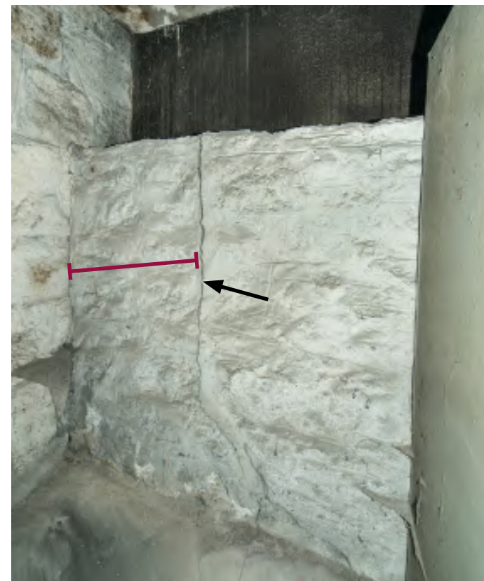
15.4: Detail of interior at west end of 1899 addition. The arrow points to the same crack that is shown on the exterior in 13.2. The red line marks the former entry to the 1899 open yard.
