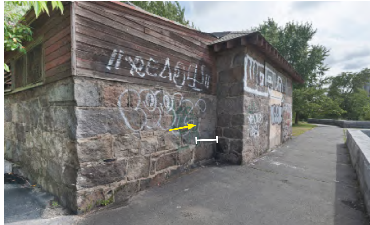
15.1: Overview of the west end of the 1899 addition and its junction with the magazine. The terrace wall in front of the building dates to 1975. The arrow points to the crack shown in 15.2. The white line indicates the position of the 1899 opening that led into the open yard defined by the addition.
