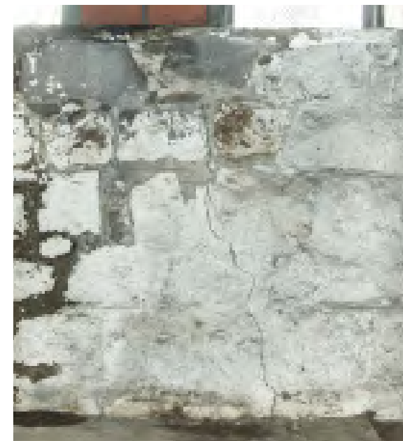
19.6: Detail of south wall (18.1) showing the crack discussed in the engineers's report that extends through the full thickness of the wall.
