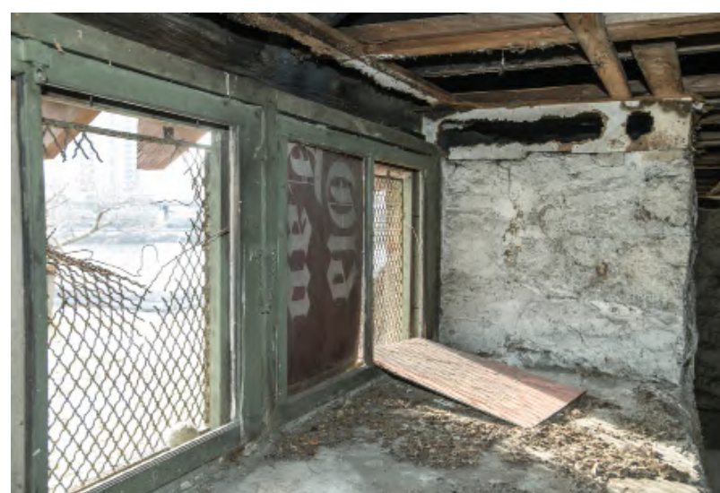
19.5: Detail of south wall (16.2) showing window set within the section of wall that was cut away in 1899 for the windows. The top of the wall has been parged with cement mortar to provide a level surface for installing the window frames.
