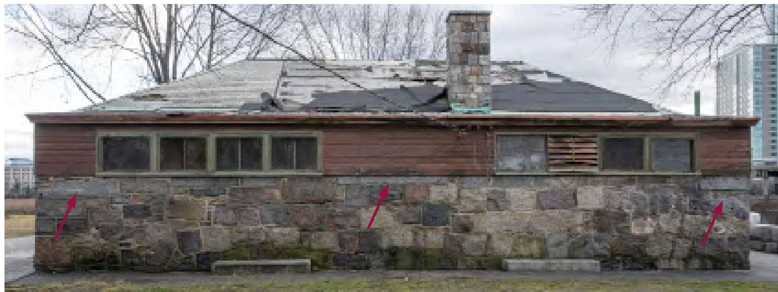
13.3: North elevation of 1899 addition. The wood siding and roof were added in 1918. The chimney was added in 1954, as was the protective screening on the window sash. Coursing of the stone is more irregular than the 1818 coursing of the south facade. Most of the stones are similar to the 1818 magazine stones in their range of color and surface texture. Most were probably salvaged from the interior partition of the magazine that was removed in 1899, the stone pier, and dressed stones lying around the site. Arrows point to examples of stone that are more modern and came from other sources. Most of slate on this pitch of the roof is missing or severely damaged.
