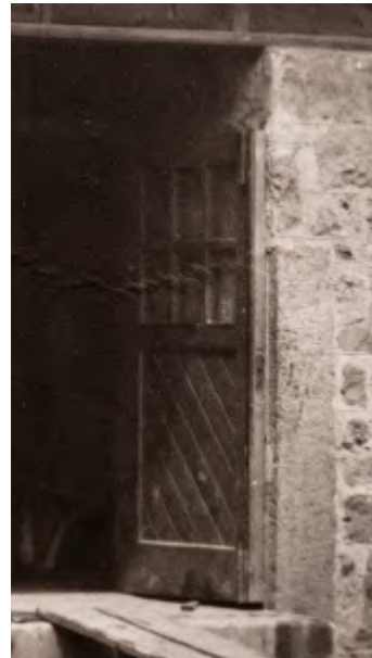
9.2: Detail of 8.1 showing the detailing of the 1918 door with a matched boarding in the panel set at on a diagonal. The original 1818 dressed granite door jamb has been reset to frame the entry.
