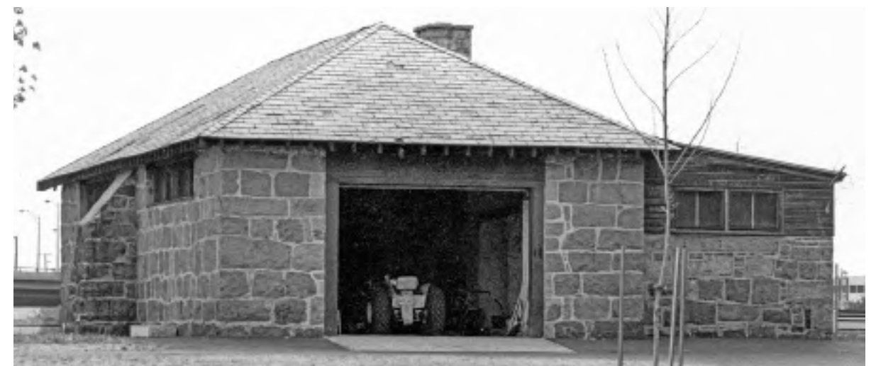
9.5: Photograph dated 1976 of the east end of the magazine showing the door opening as widened to 13' 8" in 1954. It appears to have an overhead door rather than the doors shown in the 1954 drawings. Note that the grade around the building has been raised to about half way up the first course of stone. The stone chimney has been added, along with a pair of windows at the end wall of the addition, as per the 1954 drawings.
