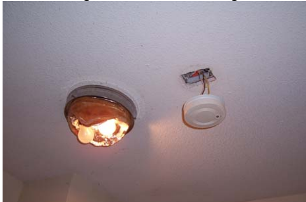
705 Development, Scattered Sites Common Area - Smoke Alarm Disconnected and Light Fixture Cover Missing
