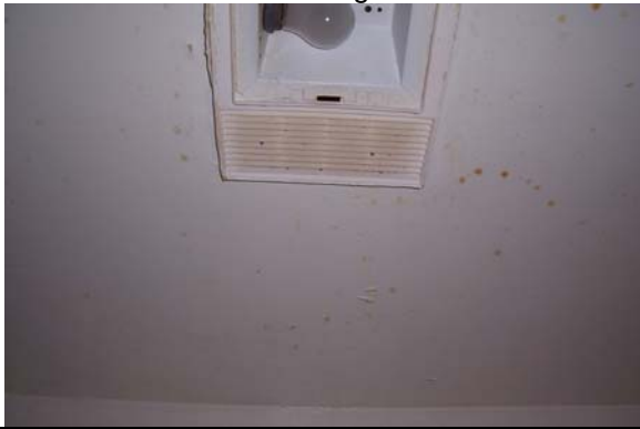
705 Development, Scattered Sites Common Area - Smoke Alarm Disconnected and Light Fixture Cover Missing
