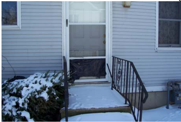
705 Development, Scattered Sites 43 Hamilton Street Storm Door Broken and Covered With a Trash Bag
