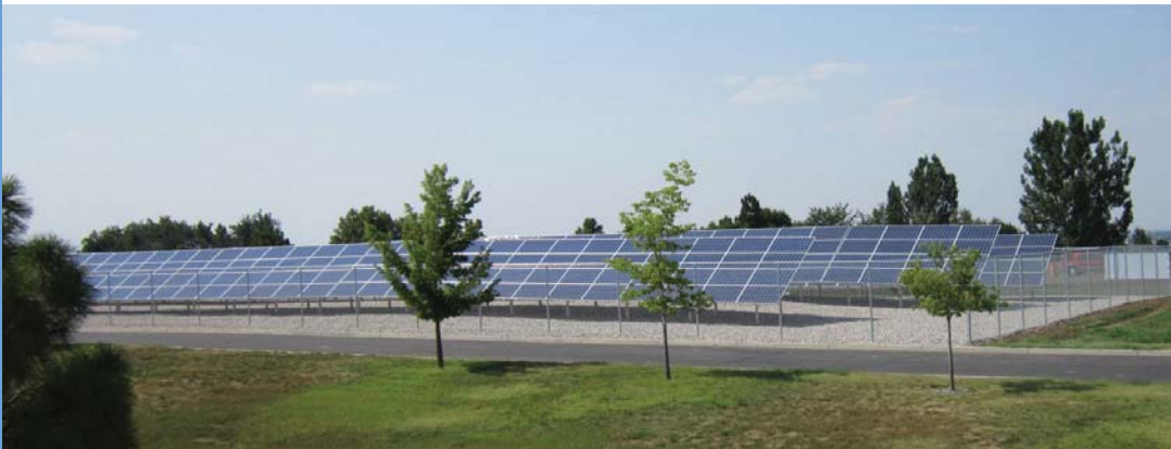
Poudre Valley REA Community Solar Farm
