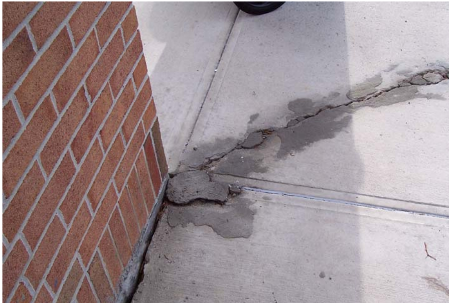
667-1 Development, Brown Memorial Court, Exterior Cracked Sidewalk Creating Tripping Hazard
