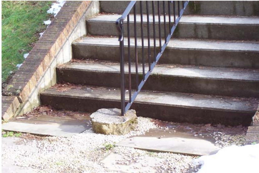
667-1 Development, Brown Memorial Court, Exterior Cracked Sidewalk Creating Tripping Hazard
