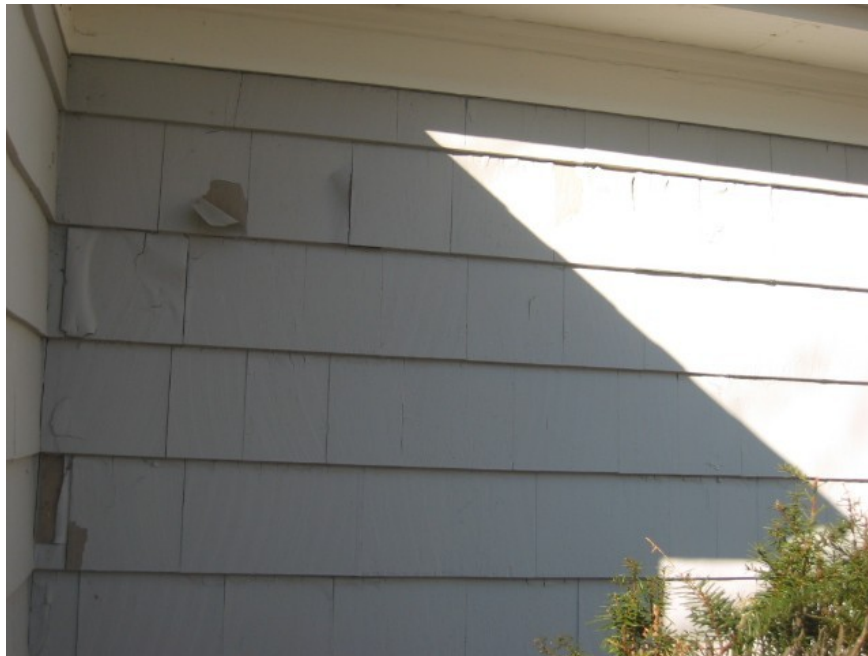
667-1 Elderly Housing Development, 14E Birchcrest Street Building Building Exterior – Paint Peeling on Siding
