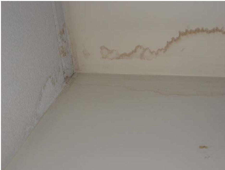
667-1 Elderly Housing Development, 15 Birchcrest Street Common Area – Water Damage on Ceiling
