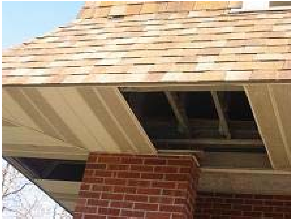
667-1 Elderly Housing Development, 15 Birchcrest Street Building Exterior – Soffit Boxes Broken in Places, Need Replacement
