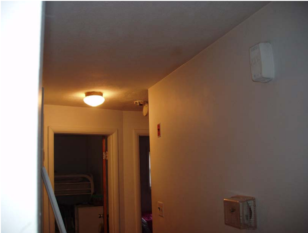
705 Family Housing Development Scattered Site, 12 Nelson Road Hallway – Cover Missing on Smoke Detector
