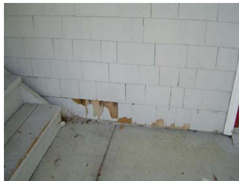
Project 667-1 Flaking Paint on Exterior Shingles
