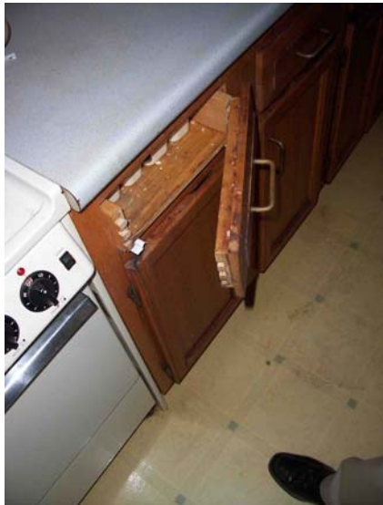
Broken drawer in kitchen
