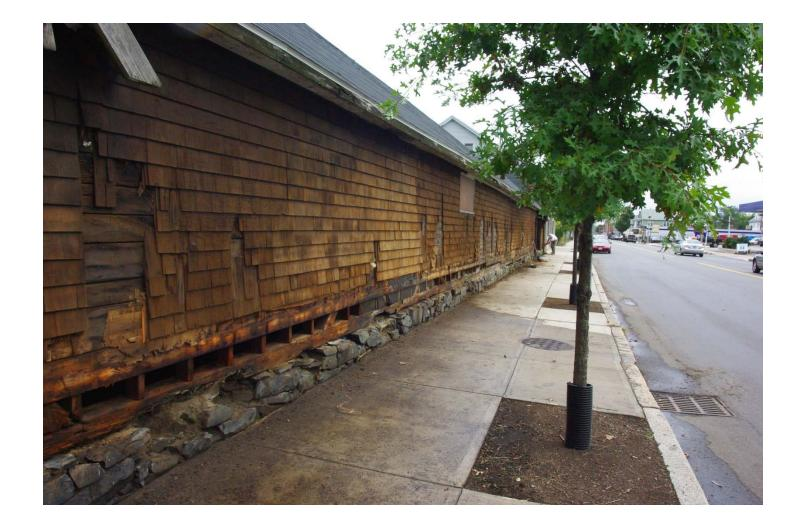
Western Ave wall at beginning of selective demolition. Note the condition of the sill beam.
