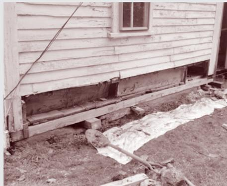
DCR replaced the rotten sill on the 1786 post-and-beam Wilbur Farmhouse in 2010, buying valuable time for the threatened structure.
