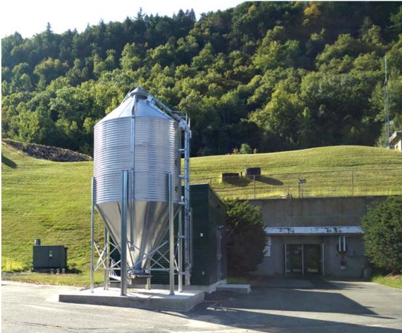
Amherst College book depository and wood pellet storage silo
