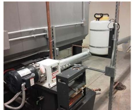
An auger injects pellets into the boiler
