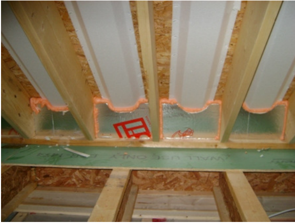
Figure 9 - Wind baffles installed and sealed in a raised heel application
