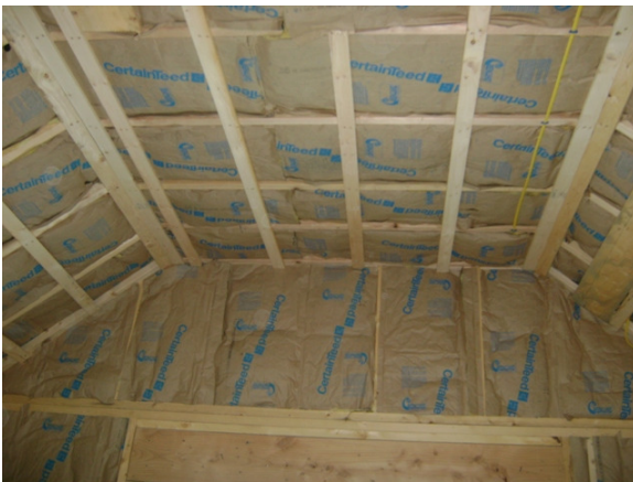
Figure 1 - Strapped ceiling insulated with fiberglass batts
