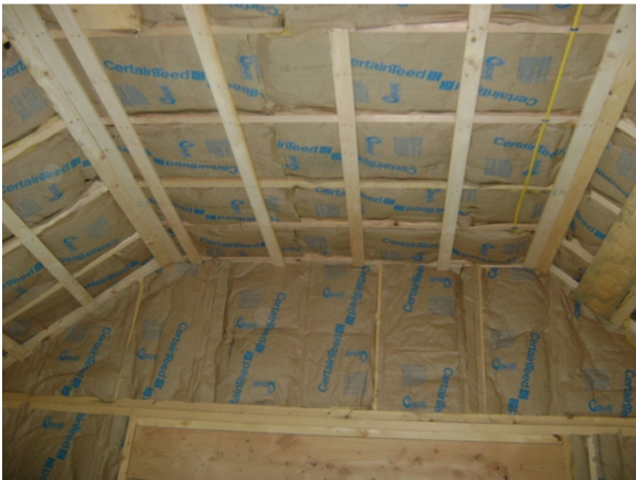
Figure 7 - Strapped ceiling insulated with fiberglass batts
