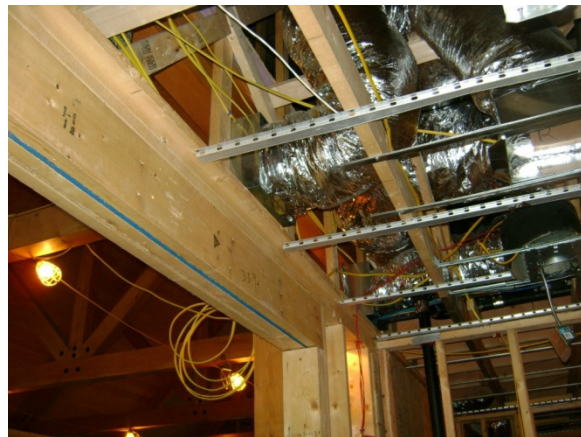
Figure 2 – Ceiling with resilient channel
