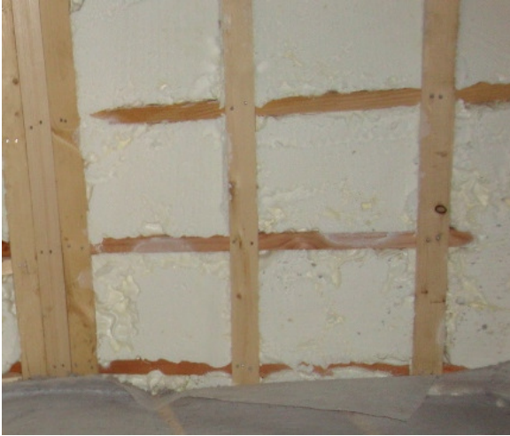
Figure 6 - Spray polyurethane foam installed in a strapped cathedral ceiling
