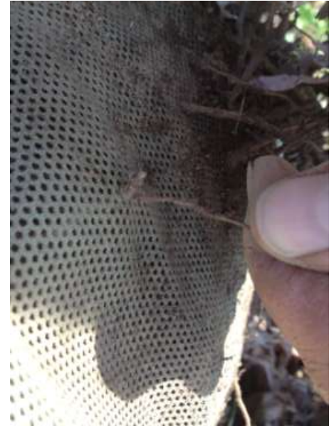
Inspecting roots growing through a fabric container. This tree was produced using the in-ground fabric method. (Rick Harper)
