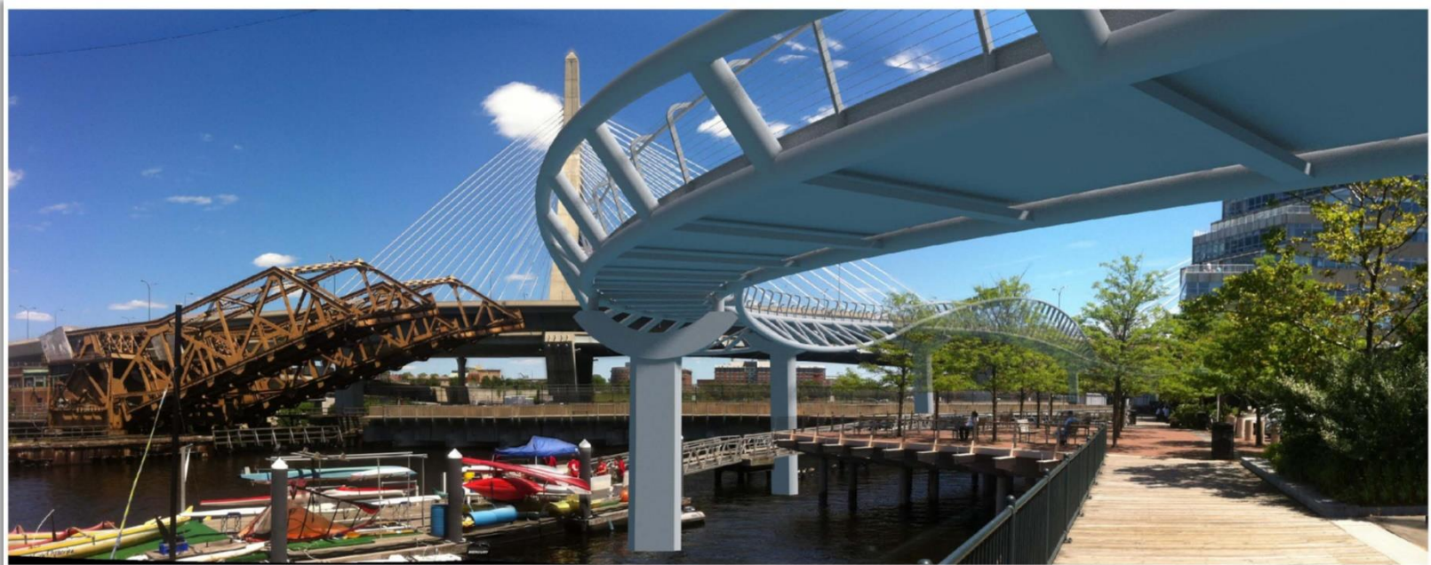
View from the seawall walkway
