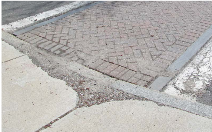
Crosswalk ramps are deteriorated.
