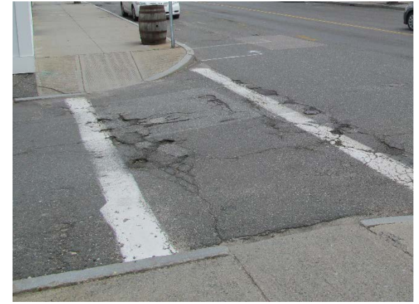
Crosswalk pavement is deteriorated.
