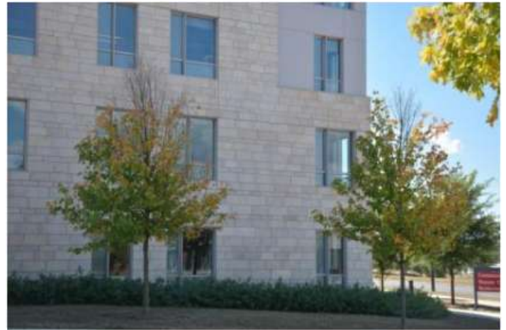
Plant damage from the top down and/or the outside in is a sign of damage from drought stress.
