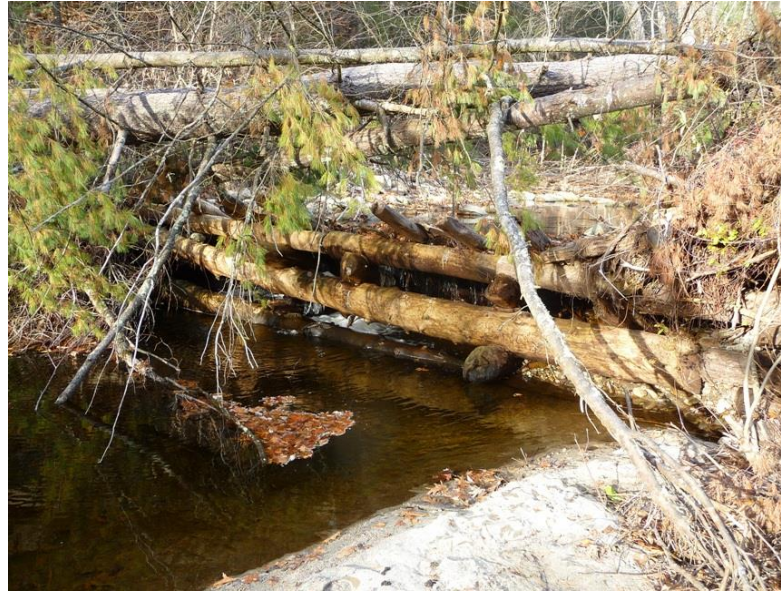
Figure 1: Timber dam, Amethyst Brook, Pelham, MA
